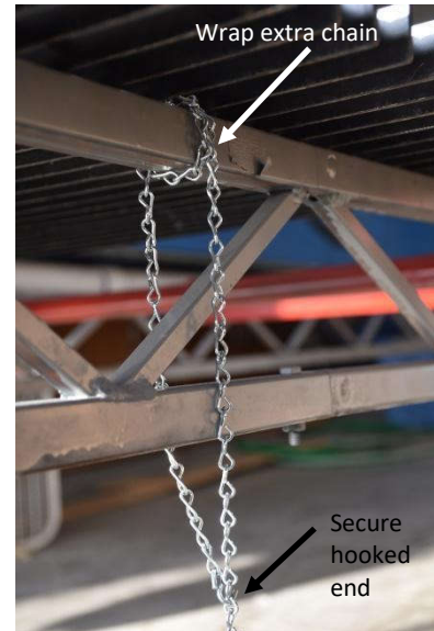
Figure 2b. Chain secured.
