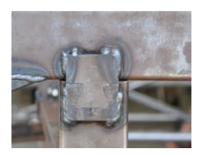
Example 15(a), 15(b), and 15(c): Prohibited tube-in-tube/sleeved connections (9.4.2.5).
