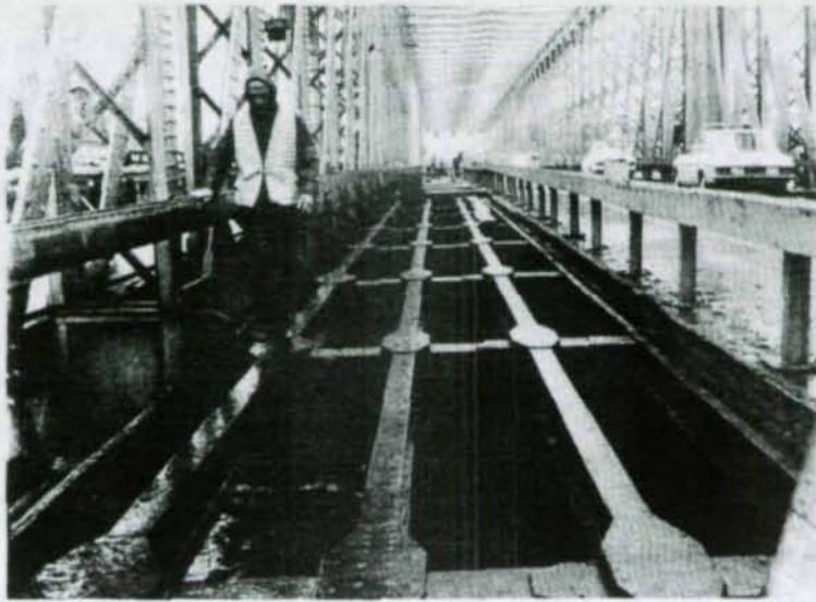
Figure 2: Riveted bridges in Rotterdam, where injection bolts were used to replace faulty rivets.
