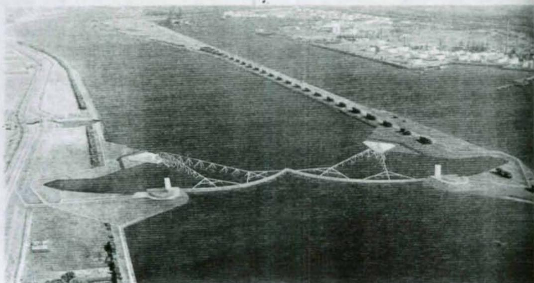
Figure 5: Artists impression of the new storm surge barrier called: "Maeslant kering". The width of the waterway is 360 meters; the height of the wall is 22 meters, and the length of the arms is 237 meters.
