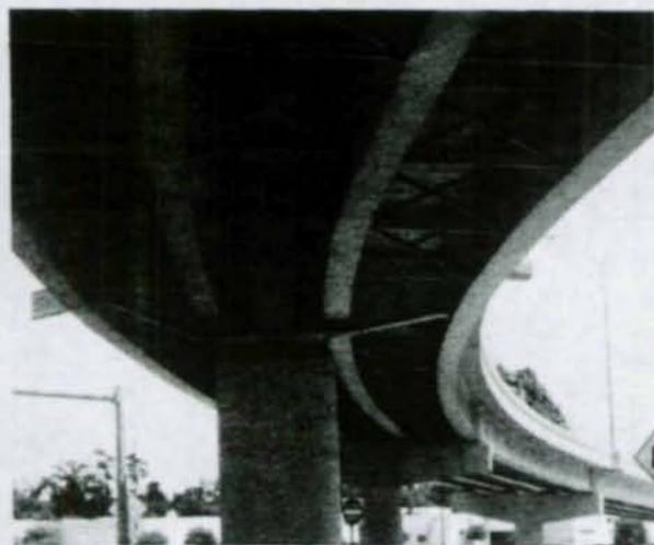
Figure 1 Connection Between Integral Steel Cap Girder and Concrete Pier
