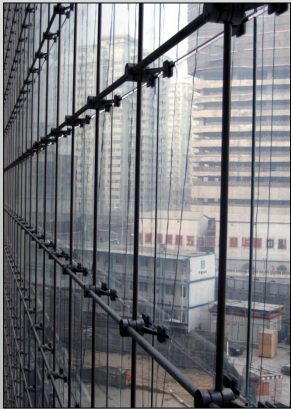
Cladding support, fittings & fasteners
