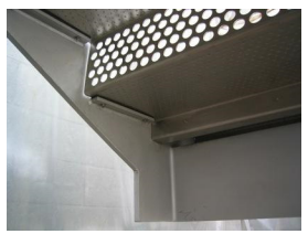
interior stair, 304L
