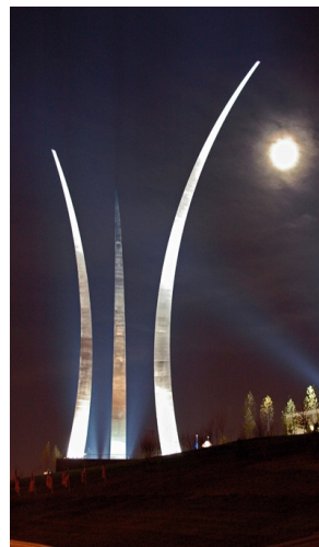
US Air Force Memorial welded 0.75 inch plate
