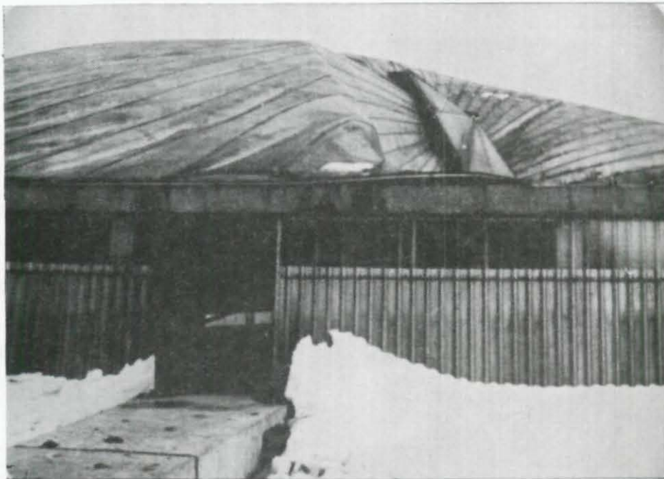
Fig. 10. View of water tank cover at Bradford, England, after failure under exceptional snow load
