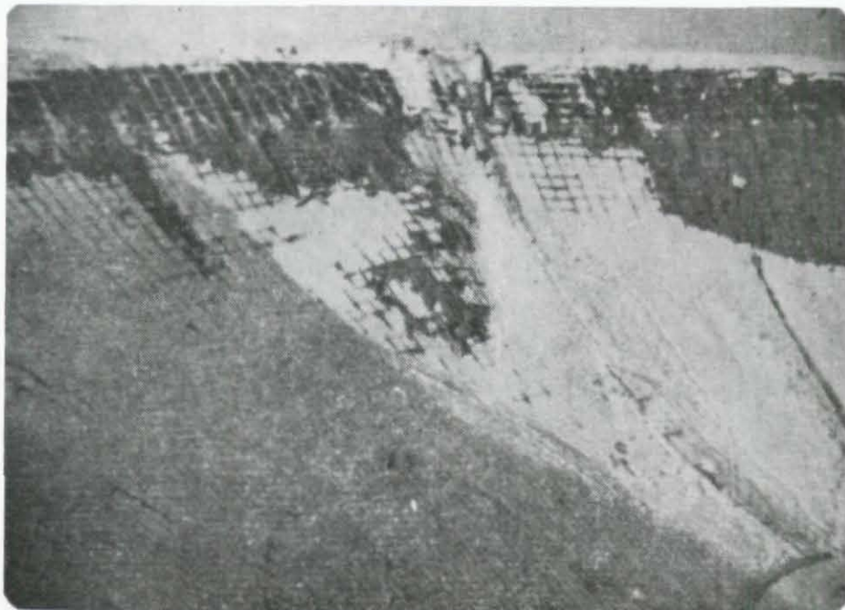
Fig. 6. View of the upper surface of Bucharest Dome after failure. Note part of cap at lower right corner
