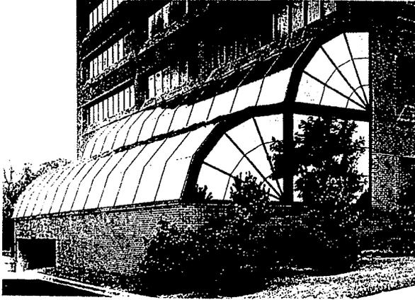
FIGURE 9 - HALF VAULT SKYLIGHT WITH END WALLS
