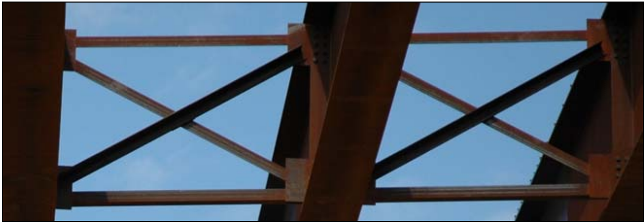
Figure 4: Single Angle X-Frame
