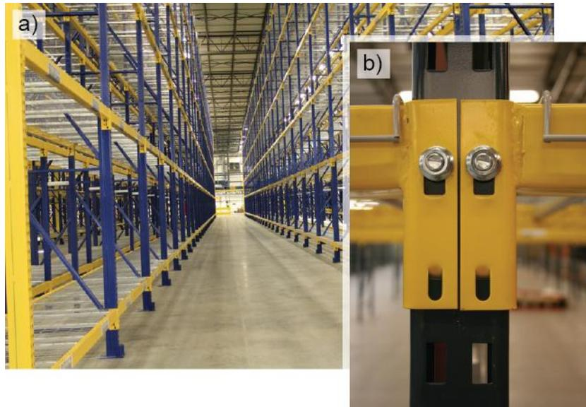
Figure 1: Storage rack a) assembly and b) shelf connection (UNARCO 2012)
