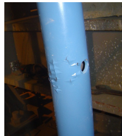
Figure 6: Yielding of Standards in Braced Frame with tie Scaffold.
