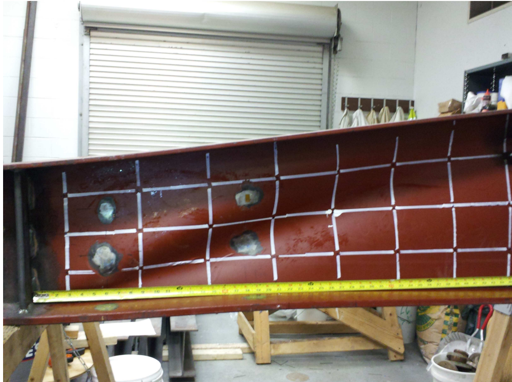
Figure 3: Tapered 4 Shear Buckling Failure
