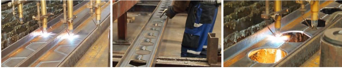
Figure 12. Production process. Left: cutting of the castellated beams. Middle: welding of the castellated beam. Right: cutting of the round openings for the cellular beams
