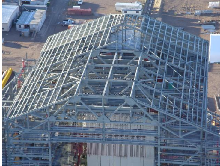
Figure 6: Modified Warren Truss in Modular Boiler Support Structure (Courtesy Bechtel Power Corporation)
