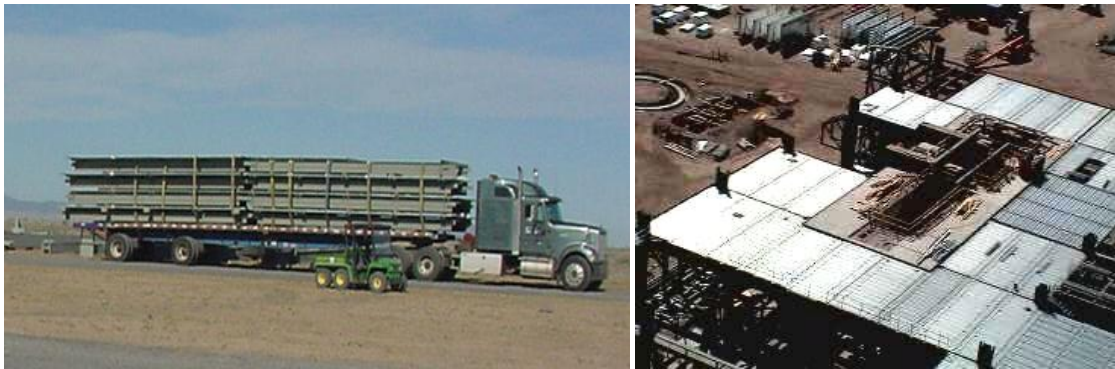
Figure 3: Stackable Modular Floor Panels in Transit and During Installation (Courtesy Bechtel Power Corporation)
