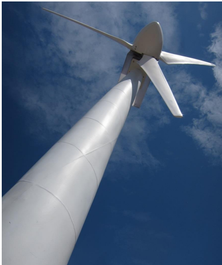
Figure 1: A small-scale, hand-welded demonstration tower completed with spiral weld geometry [Image courtesy of Keystone Tower Systems].
