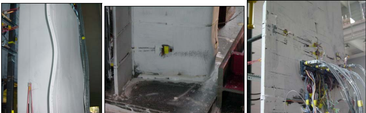
Figure 8: Column and beam-column test failure modes, local buckling at deck plate, rib and yield lines on the deck plate
