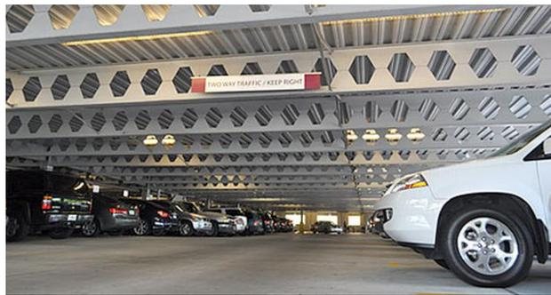
Figure 1. Application of castellated beams (Scherer Steel Structures, Inc.)
