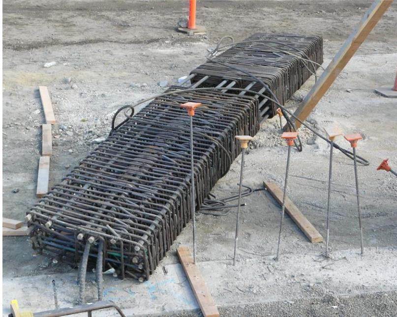
Figure 3: Collapsed column rebar cage example 1
