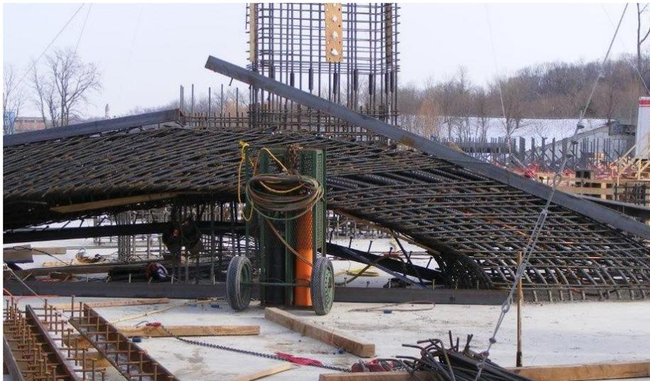
Figure 4: Collapsed column rebar cage example 2
