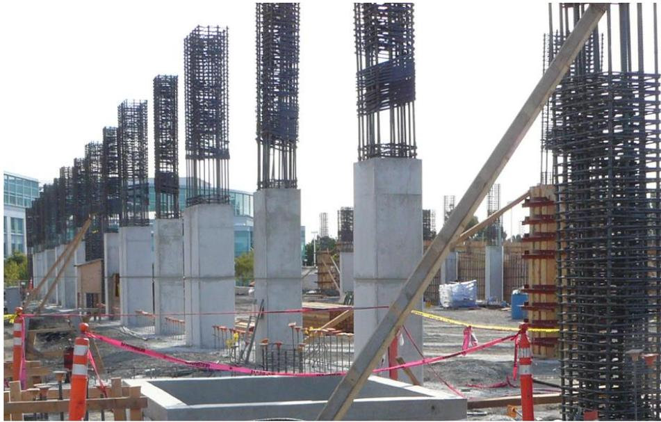
Figure 1: Column cages during construction with partial-height concrete
