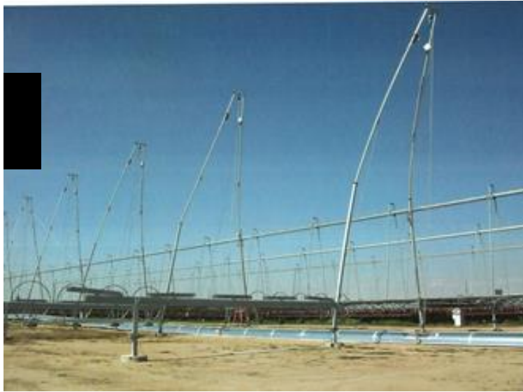
Figure 3: Post-incident photograph of bent towers
