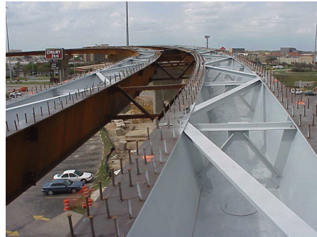
Figure 1: Bracing Systems for Twin Tub Girders During Construction
