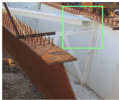
Offset in strut/internal K-frame
