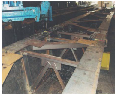
Excessive use of internal K-frames.
