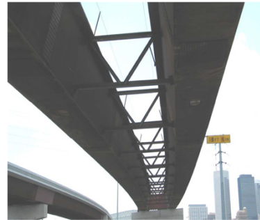
Excessive use of external K-frames.
