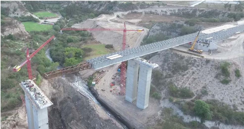
Figure 2: Bridge erected with the incremental launching method
