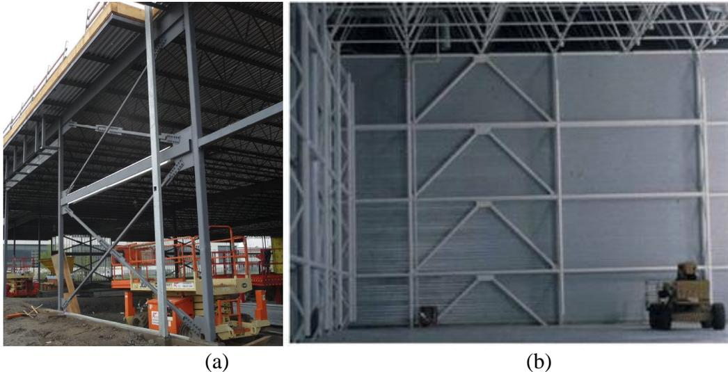
**Figure 1.** MT-BFs in single-story, steel buildings (Imanpour et al. 2016) (a) 2-tier X bracing (b) 4-tier chevron bracing (Imanpour and Tremblay 2016).
