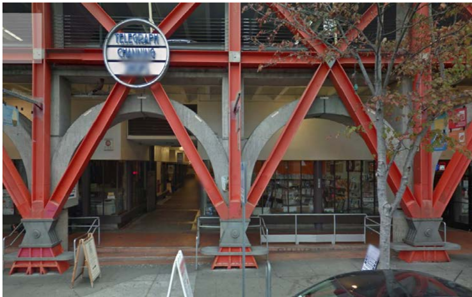
Figure 2: Actual Boundary Conditions - "pin" connection at column base in Berkeley, CA (source: maps.Google.com)
