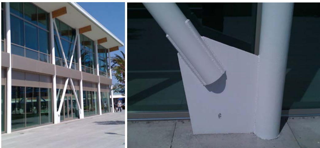
Figure 3: Actual Boundary Conditions –gusset plate for bracing members at the Ferry Building in Oakland, CA
