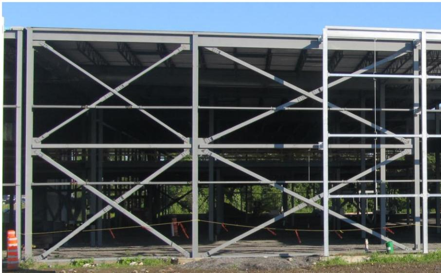
Figure 1: Typical steel single-story industrial building with a multi-tier configuration
