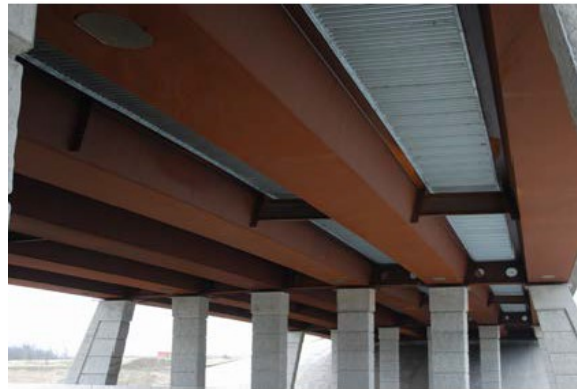
Figure 2 - Shallow Tub Girder System from Waco District
