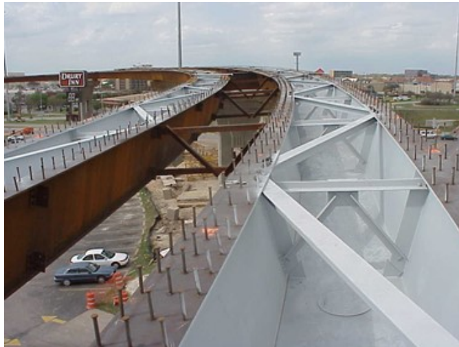
Figure 1 - Bracing systems in twin tub girder during construction
