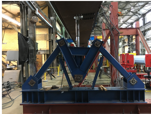
Figure 10 - Gravity Load Simulator (GLS) during test
