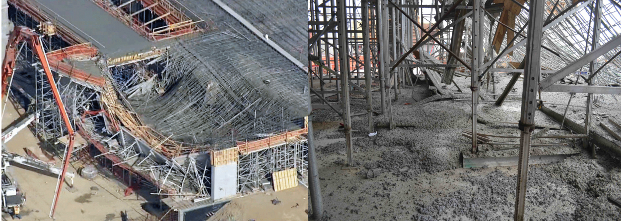
Figure 1: Photographs of Collapse, Ariel View and Below Level of Collapsed Shoring
