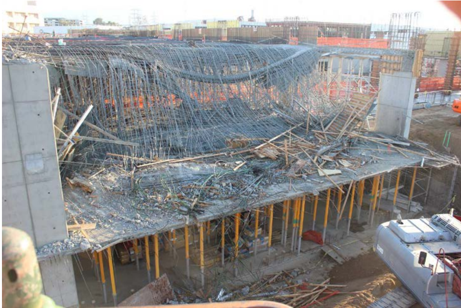
Figure 1: Partial garage collapse during concrete pour
