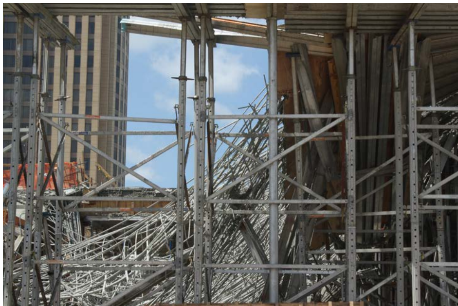
Figure 2: Close-up of aluminum shoring/forming system
