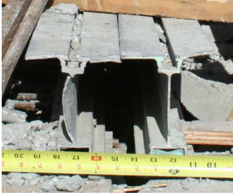
Figure 6: Aluminum stringers; left example shows web fracture and buckling
