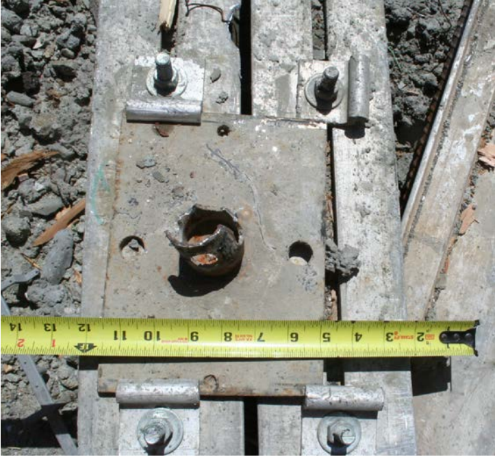
Figure 7: Offset in stringer loading
