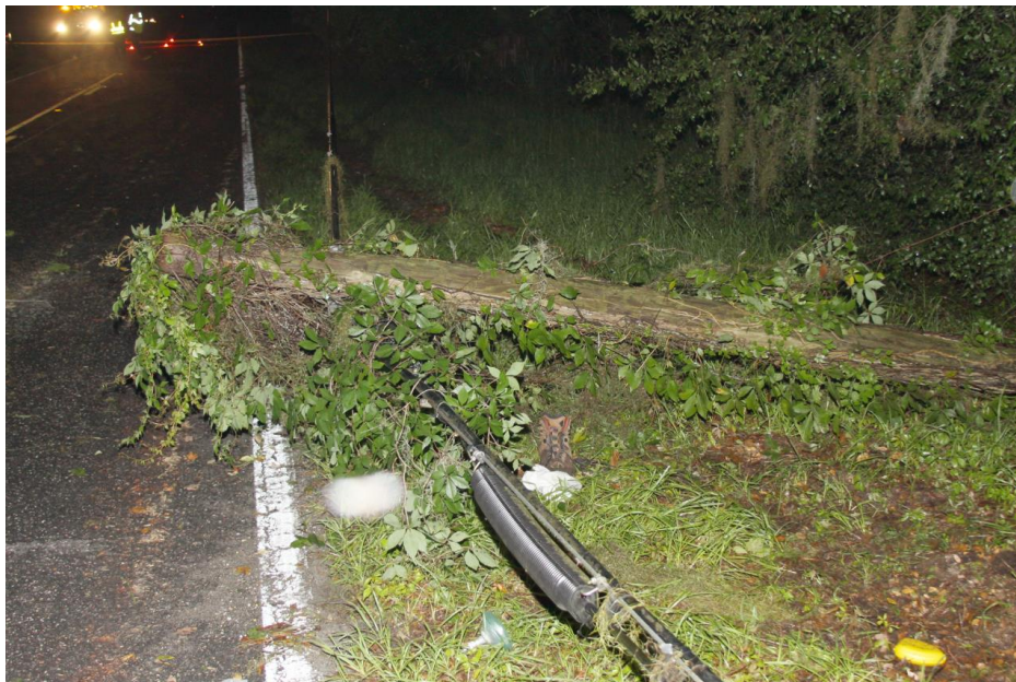
Figure 3: Failed utility pole
