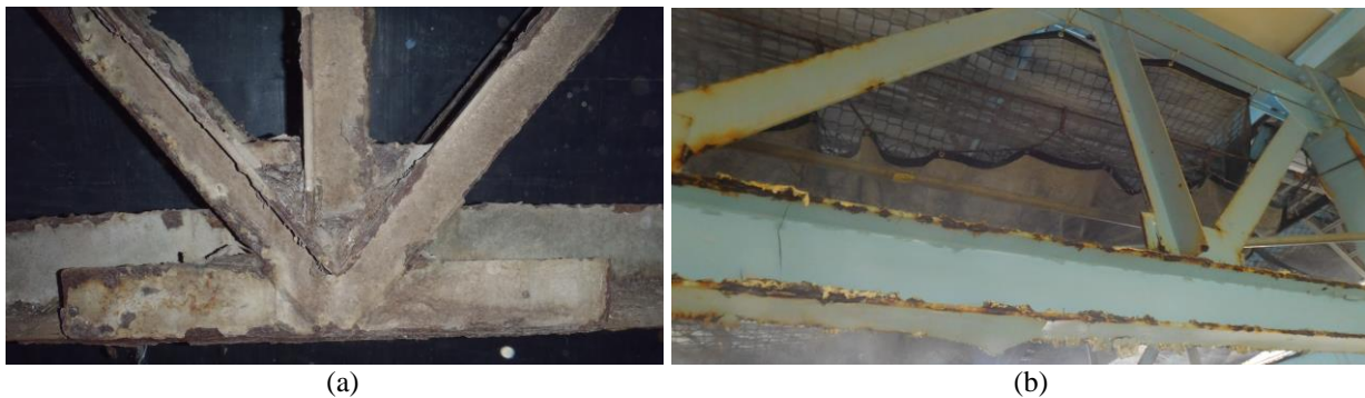
Figure 1: Examples of Corrosion in Steel Roof Trusses in Two Different Industrial Facilities
