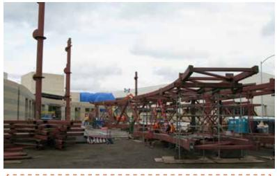
The walkway walls, floor and roof were designed as full trusses with the shop-fabricated roof and floor segments assembled on the ground at the site. Wall elements were field-welded to the floor and roof segments and then erected.
