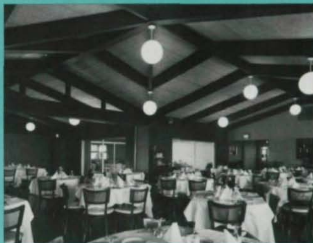
Dining area is unencumbered by columns. Simple steel space frame is painted redwood color.
