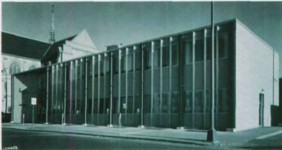
Completed building has a monochromatic color scheme: buff-colored brick, raffia-tan panels and chocolate-brown steel columns.
