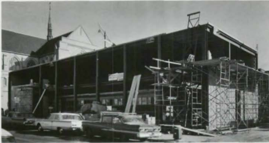
The older building is visible behind the two-story-high steel columns which support the new building.
