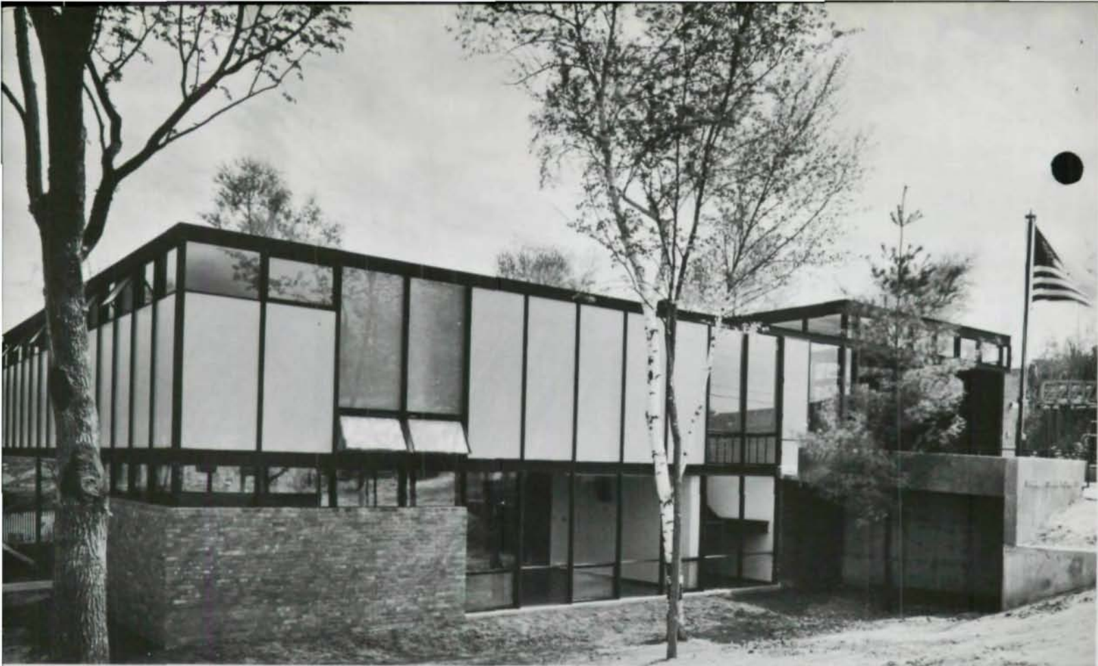
Cedar Rapids Fire Station #8 shows what can be done to achieve style, utility and economy in a modern firehouse located in a new residential area. Exterior steel is painted dark brown, and Fiberglas panels are gold-colored.
