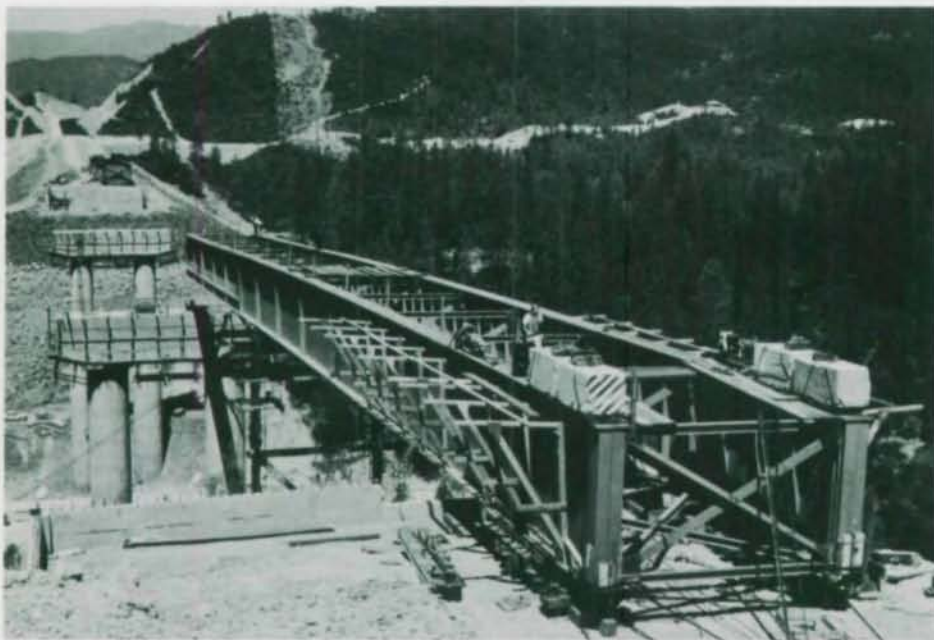
A pair of 305-ft end-span girders rolls into position. The long girders were assembled at the bridge approaches, then moved on a nest of steel rollers.
