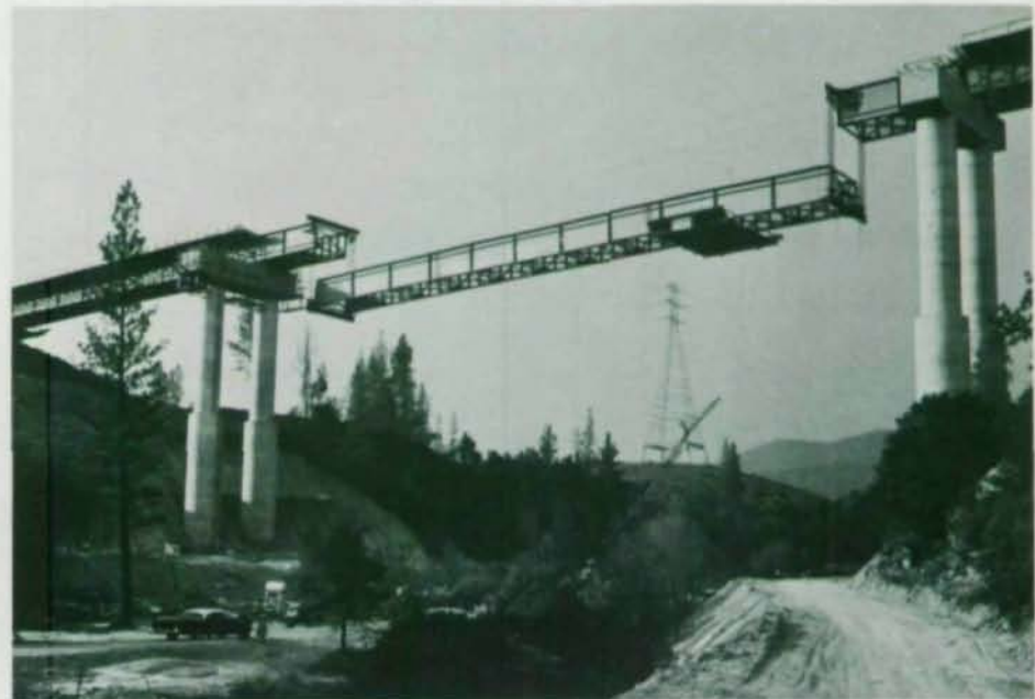
The 200-ft suspended span is hoisted into place by lead-line pull engines and a series of wire rope lifting falls.
