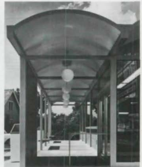
Square steel pipes and rolled sections were used as the frame for the Burger Boy Food-O-Rama store in Columbus, Ohio.
