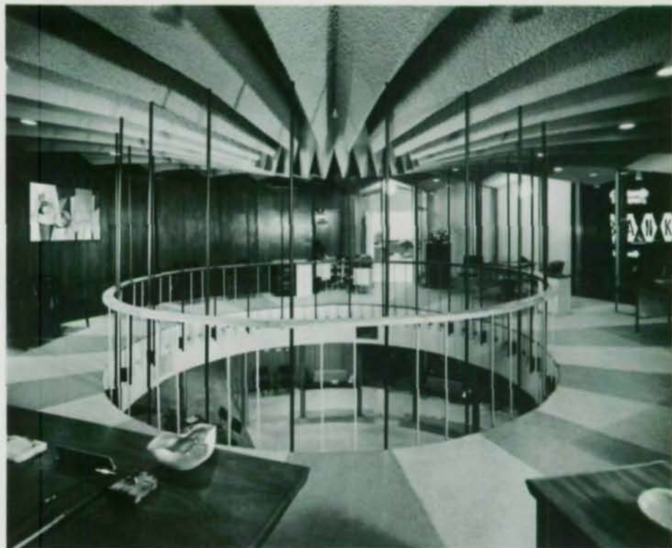
Pleated ceiling of the circular section is gold-colored acoustic plaster. Tie rods support the railing.
