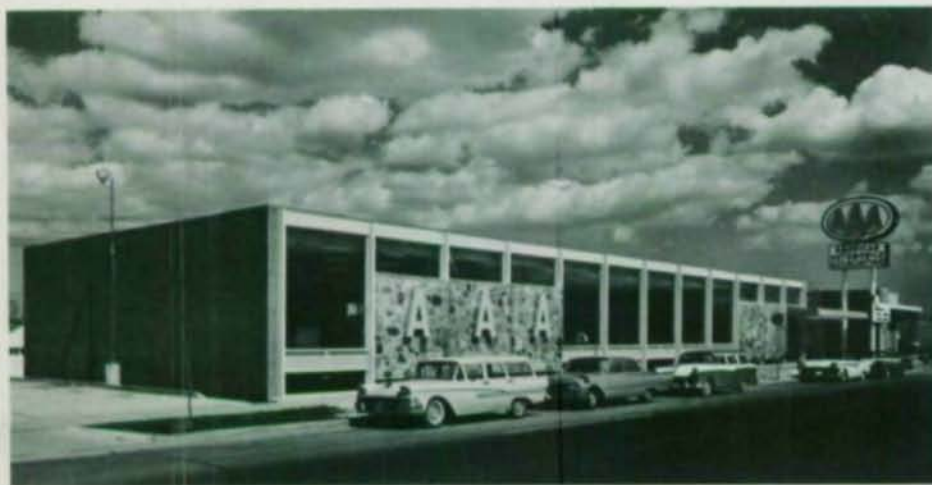
The use of exposed steel tubes for the Wisconsin Division of the American Automobile Association formed an interesting facade, and, according to the architects, was very economical.
