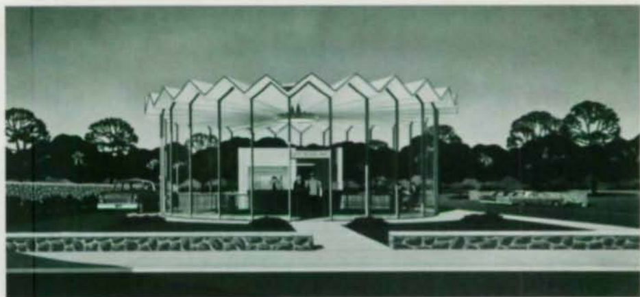
The branch office building for the Union National Bank, Youngstown, Ohio, is a circular structure framed with tubular columns. The thin steel folded plate roof spans 50 ft with no need for interior supports.
