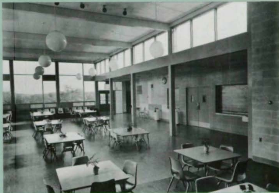
The exposed steel framing for the Pioneer School utilizes specially welded channels that not only meet load specs but require little or no finishing material as well as permitting broader, better supported fenestration.
