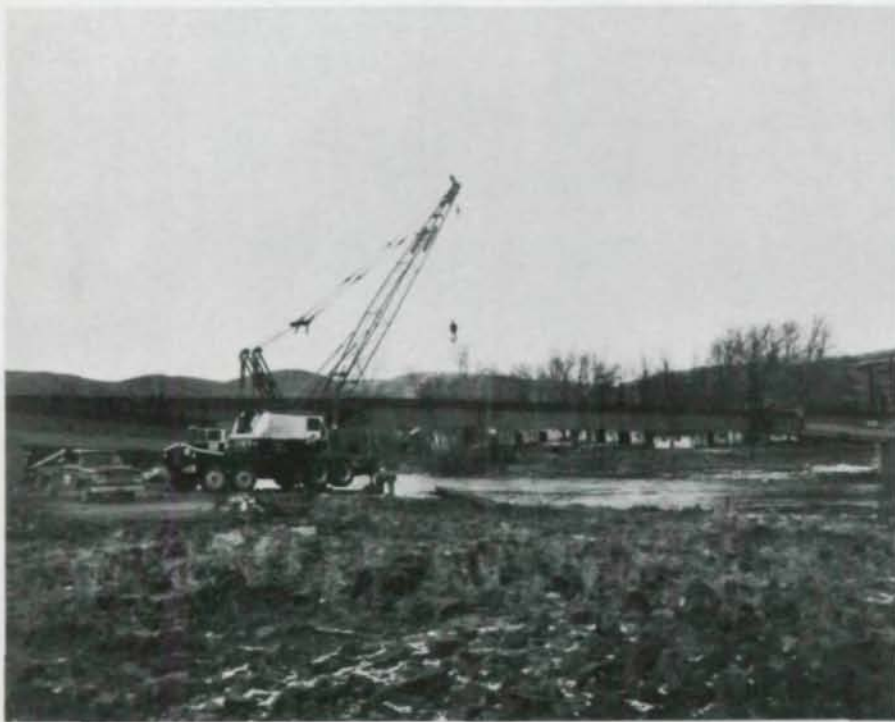
The lateral stability of the rugged delta girder makes it easier to erect than conventional plate girders and precast concrete girders.
