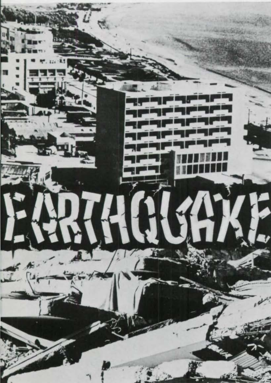
The Immeuble Consulaire, an eight-story office and apartment building housing 300 people in Agadir, is shown before and after the earthquake. A modern architectural facade proved to be no substitute for inadequate reinforcing at joints of walls and floors. The building was not braced to resist the lateral forces generated by the shock. Note the stack of successive floor slabs and precast beams.
