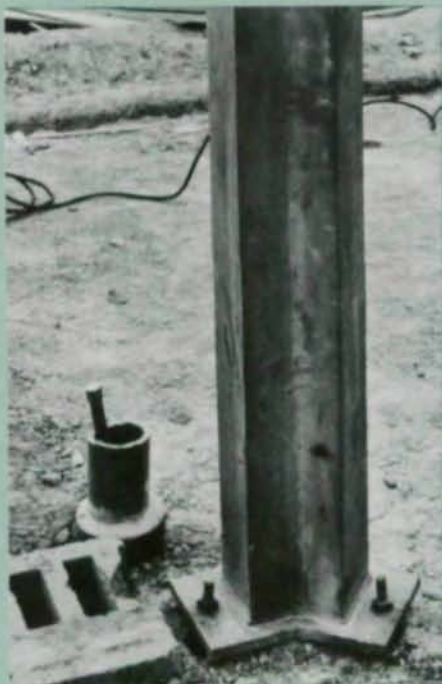
Welded corner supports on a 45-degree angle were designed to establish a gentle curve where halls change directions.
