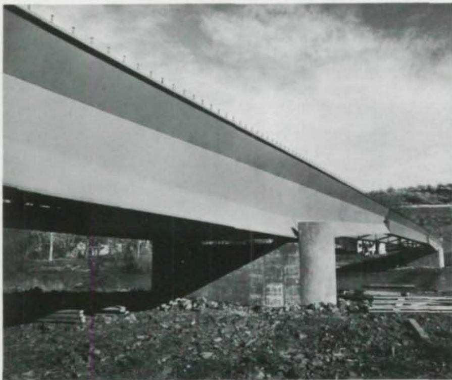
The 240-ft main span of the Parker Bridge near Yakima, Washington, comprises two 60-ft double delta cantilevers carrying a 120-ft suspended span.
