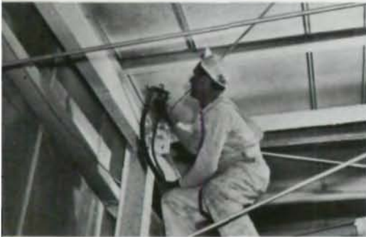
Application of Albi-Clad spray-on coating
