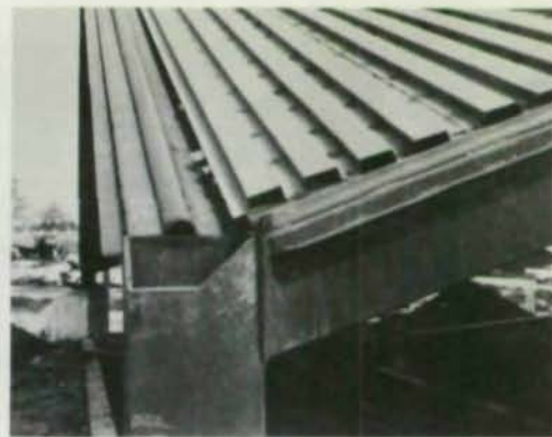
View from outside corner (left) with ridge and edge beams in place. The stub corner columns are cut off at an angle to receive drain scuppers. Corner view (right) without overhang showing deck welds and general arrangement. Half-round pipes on edge beams are used for welding attachment of roof.
