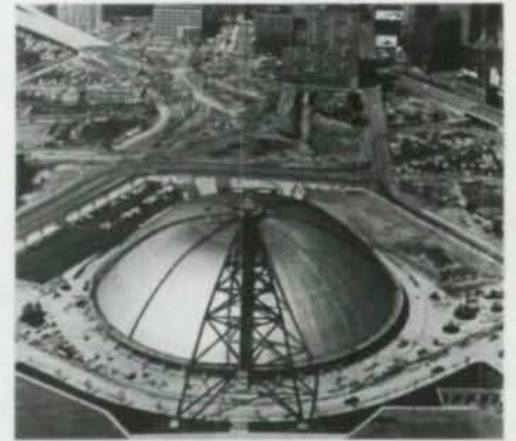
Pittsburgh Auditorium Mitchell and Ritchey, Architects
