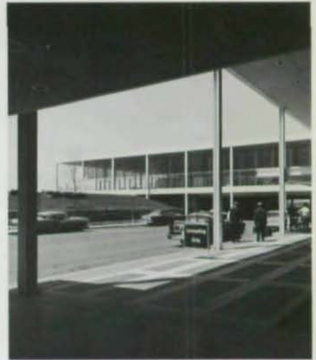
Tulsa Terminal Building Murray-Jones-Murray, Architects
