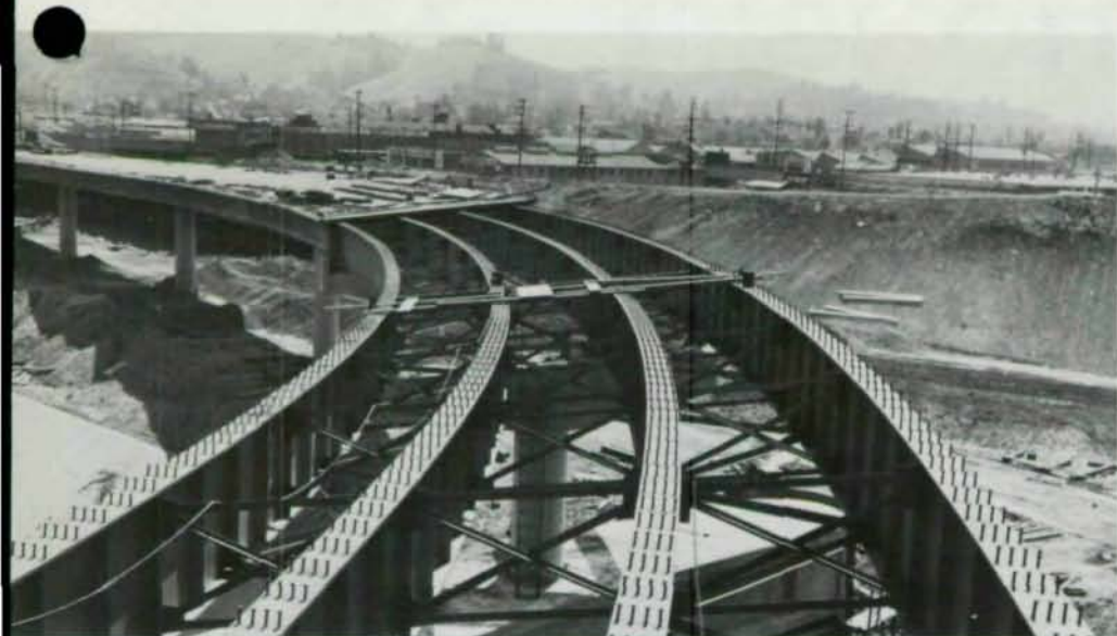
Photographs show the curved steel girders being fabricated in the shop (below) and erected ready for the placement of the composite deck.
