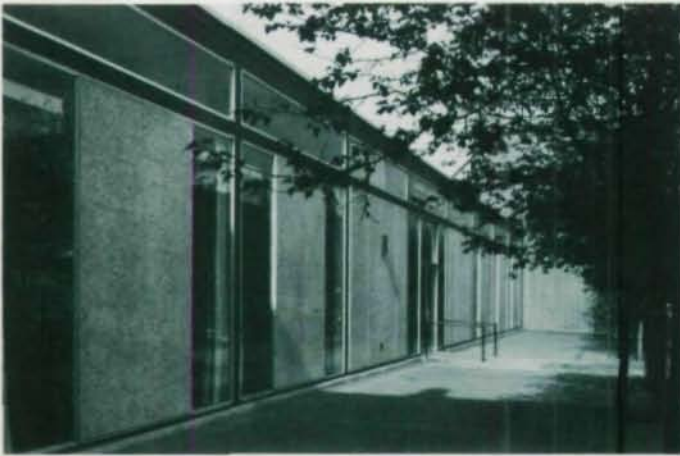
Left: The library's two reading rooms (one in foreground, the other in background at right) are separated by a low-ceilinged administrative section at left. Right: Dark areas of the library's exterior are steel painted dark green to contrast with the aluminum frames and to complement the grayish precast concrete panels.
