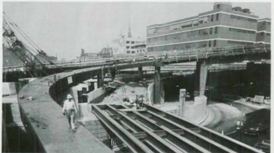
The curved box girder supports a roadway ramp to the new upper level of the Port of New York Authority Bus Terminal on Eighth Avenue in New York City.
