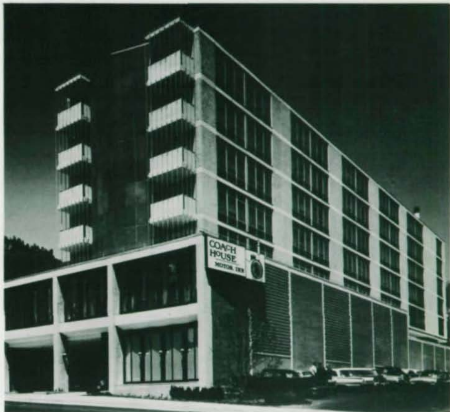
Cantilevers are expressed architecturally by curtain walls between the five upper floors and by a belt of precast units at the floor line. The column bay is emphasized by a vertical panel of precast units in which the aggregate is exposed.
