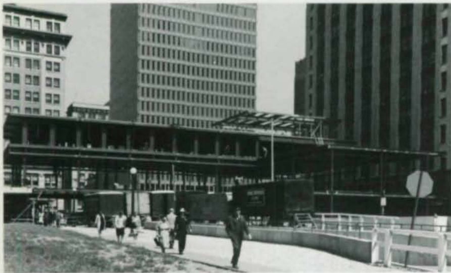
The completed structural frame work blends nicely into the background of the Blaustein Building designed by Mies van der Rohe.
