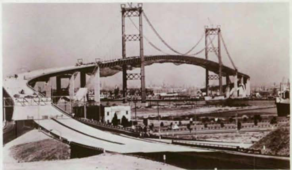
The Vincent Thomas suspension bridge spans the main channel of busy Los Angeles Harbor from Terminal Island to San Pedro with a 1500' main span and two 506.5' side spans. Including the steel plate girder approach spans, the bridge totals 6,062' long.
