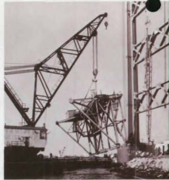
Valuable time was saved by moving the "creeper" platform, used to erect the first tower, across the channel to the second tower by means of a 125 ton floating crane.
