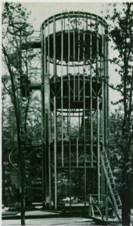
With only five levels (one below grade) and one room in diameter, this unusual, round house combines Japanese, Finnish, and American ways of relaxing. Steel-framed structure is covered with redwood.
