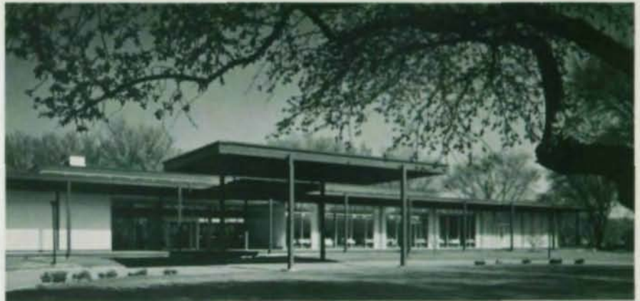
ABOVE: West elevation looking toward entry canopy. BELOW: Arcade and entrance on west elevation of building. East entrance is identical except for the main canopy at right. Formal dining room is directly behind draperies.
