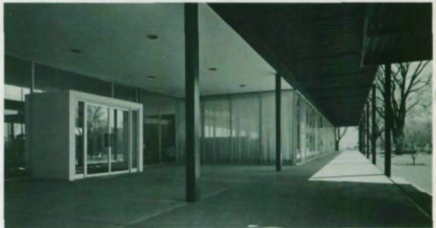
MAIN LOBBY: Canopy over bar is constructed of steel tubing with walnut edging. Acoustical ceiling is hung from the steel tubing. In background are walls enclosing the central core containing the kitchen and bathrooms.
