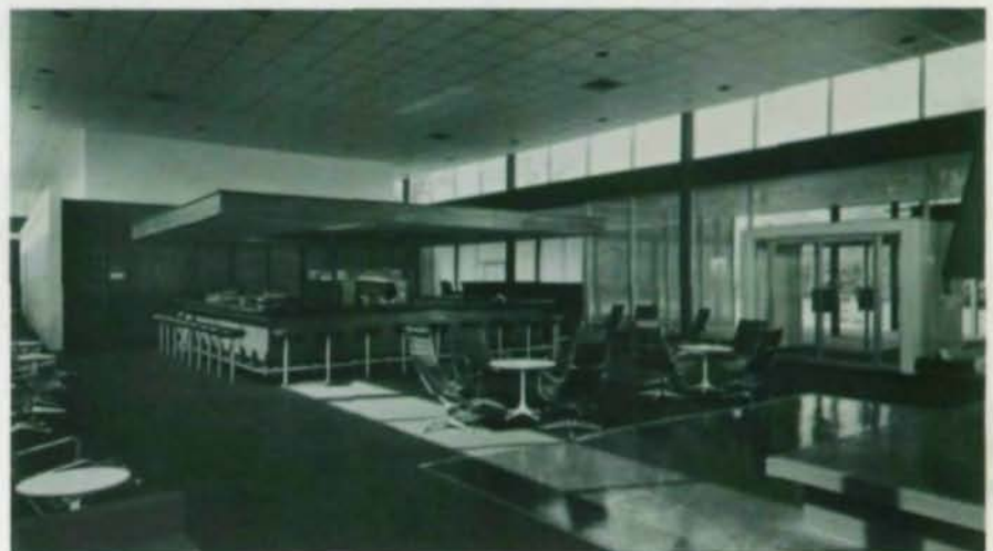
MAIN LOBBY: Canopy over bar is constructed of steel tubing with walnut edging. Acoustical ceiling is hung from the steel tubing. In background are walls enclosing the central core containing the kitchen and bathrooms.
