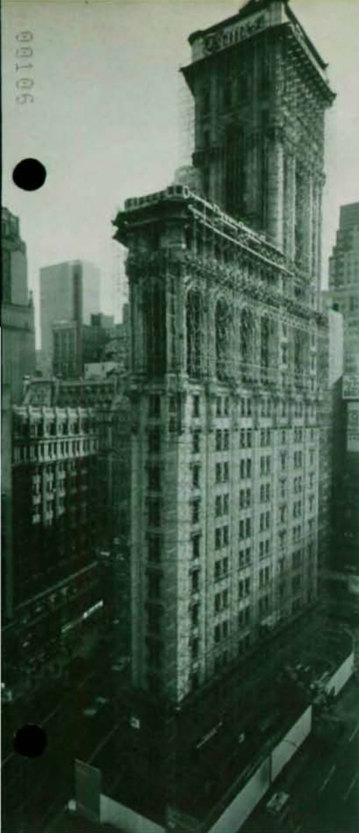
Original, 60-year-old Tower was too valuable to demolish; New York zoning restrictions would have limited any new building on the same site to only 10 or 12 stories.
