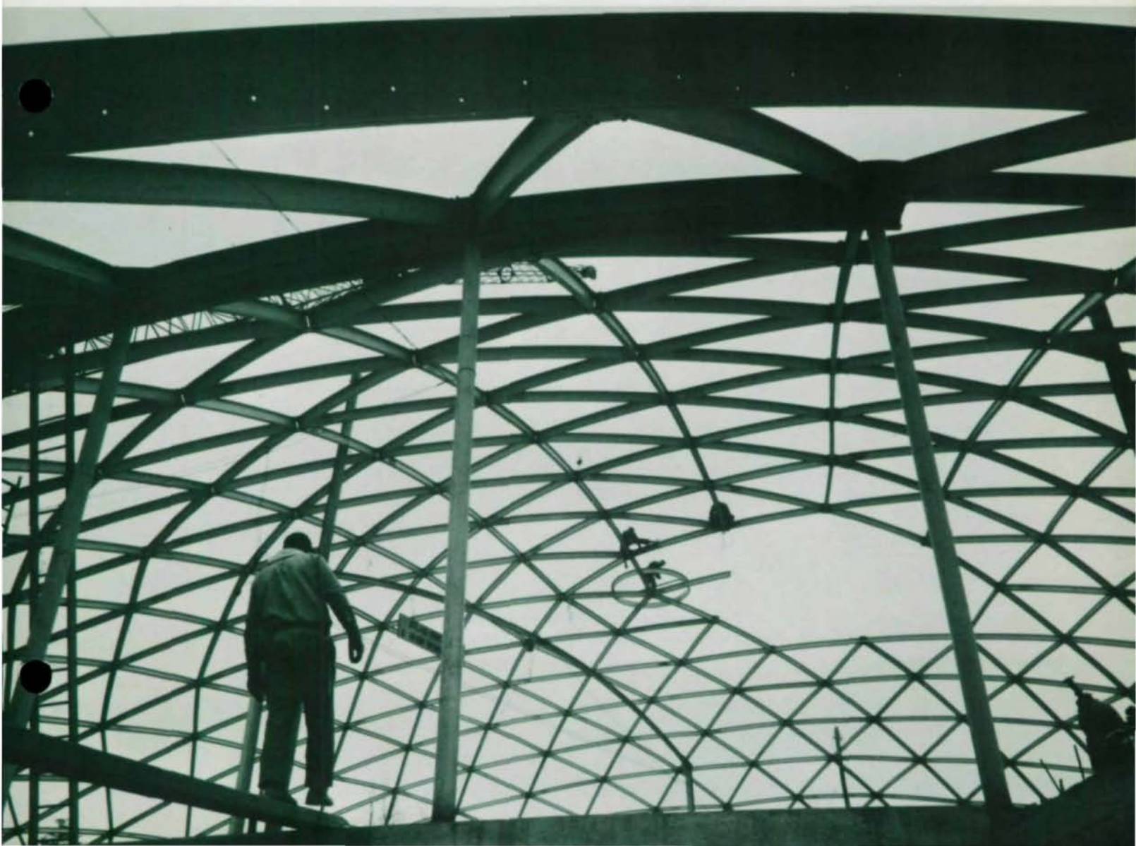
A Study in Patterns as the 8B10 Geodesic Grid Members Near Final Erection.
