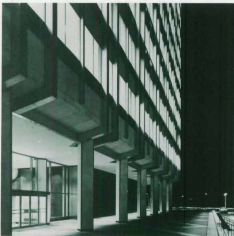
Outward Cantilevering Provides Easy Transition from Building to its Foundation.
