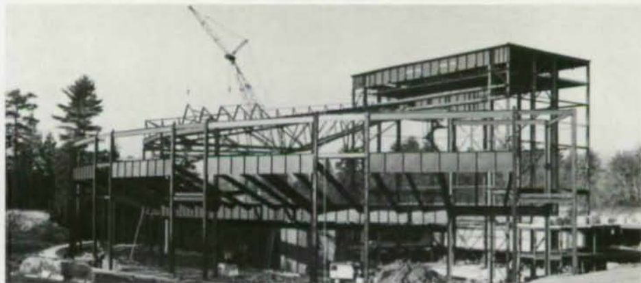
Steel frame was designed to aid acoustics. Six steel trusses, each 126 ft long and 16 to 25 ft deep, fan out from a huge proscenium girder to form a pleated roof.
