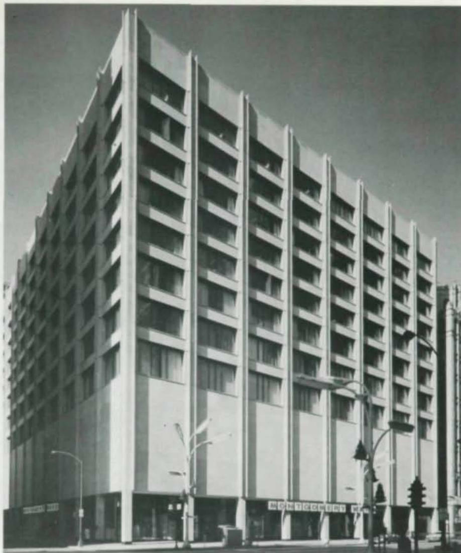
Montgomery Ward store reflects lightness and vigor of its 75-year old steel frame.
