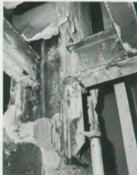
Detail of original beam and column framing. Note seats, simplicity of framing in both directions, and absence of wind moment connections.
