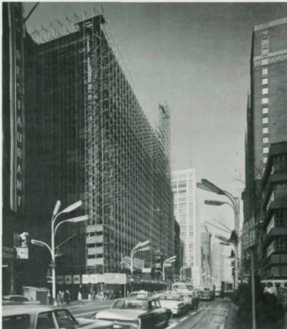
Renovation of the eleven-story Fair building, built in 1891, began in the Summer of 1964. The original steel frame was found to be in practically "mint" condition — was re-used without major reinforcing.
