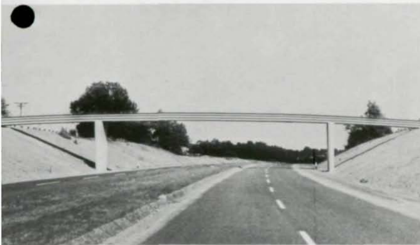
▶ Niles Street Pedestrian Overpass, Leominster, Massachusetts A clean, simple profile makes this plate girder bridge appear light and airy when viewed from the roadway.
