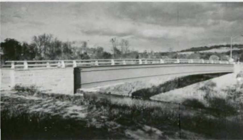
◀ Chaffee Avenue Pedestrian Bridge, Syracuse, N. Y. A welded through-deck plate girder structure. Span length is 123 ft. Access is at grade, eliminating the need for ramps.
