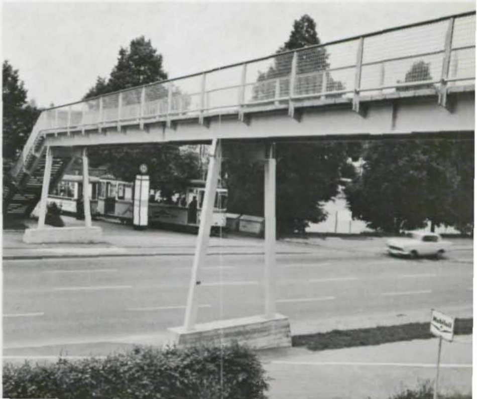
● Bridge at Killesberg, Stuttgart, Germany Girders below the deck and simple, open railing permit unhampered view on either side.
