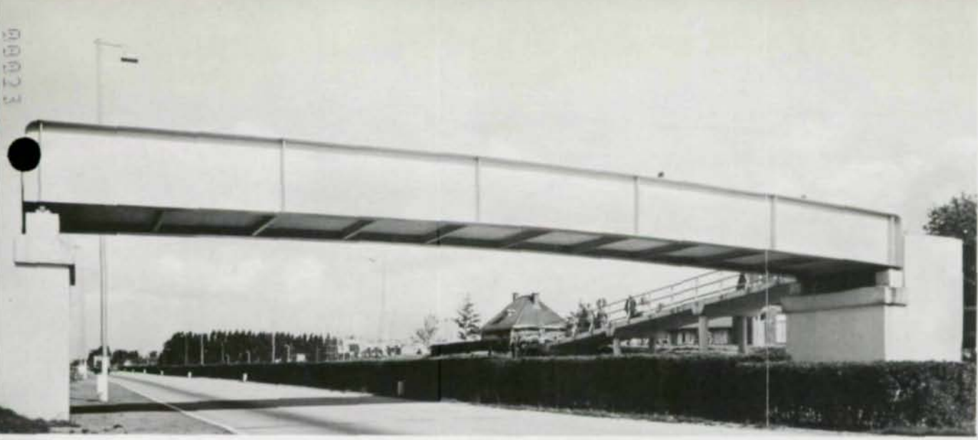
▲ Bridge near Dortrecht, Holland This through-deck plate girder bridge spans the roadway without intermediate piers. Tops of girders are at normal handrail height to permit pedestrian visibility at the sides. Access ramps are at right angles to the main span.
