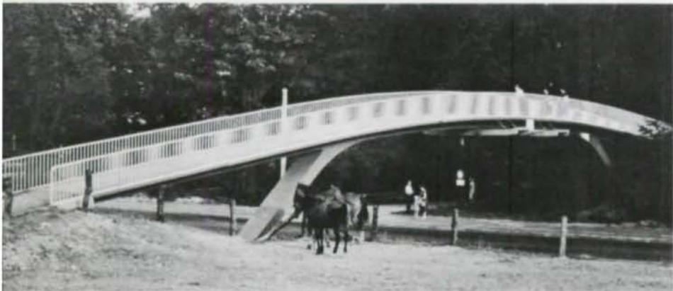
◀ Footbridge in Westfalen Park, Dortmund, Germany This graceful span is designed as a rigid frame. The main girder and sloping piers are hollow box sections.
