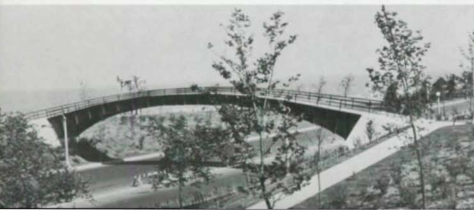
◀ Burnham Park Pedestrian Bridge, Chicago, Illinois The span length of this graceful arch bridge is 115 ft. The deck follows the contour of the arch.
