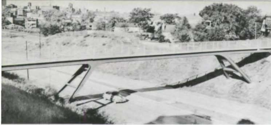
◀ Garrison School Pedestrian Bridge, Kansas City, Missouri The sloping steel piers of this rigid frame structure provide a light, pleasing appearance from the roadway.
