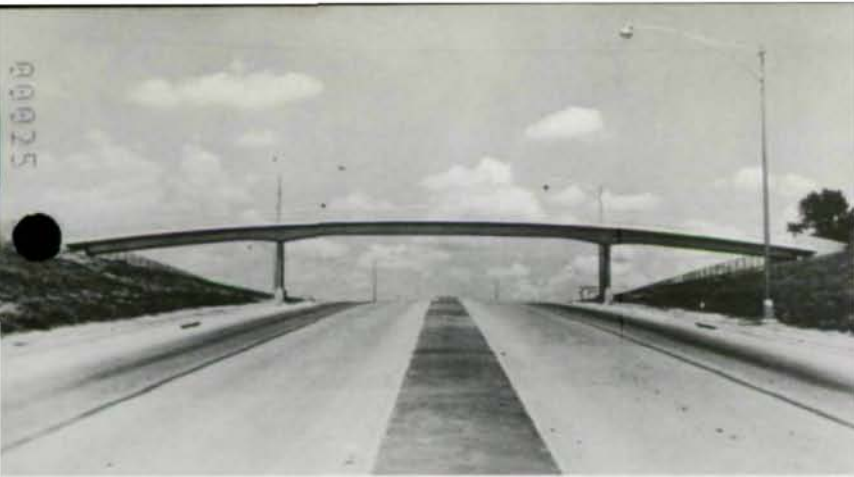
◀ Robert Street Overpass, Fort Worth, Texas Topography permits elimination of ramps or stairways for access to the bridge.
