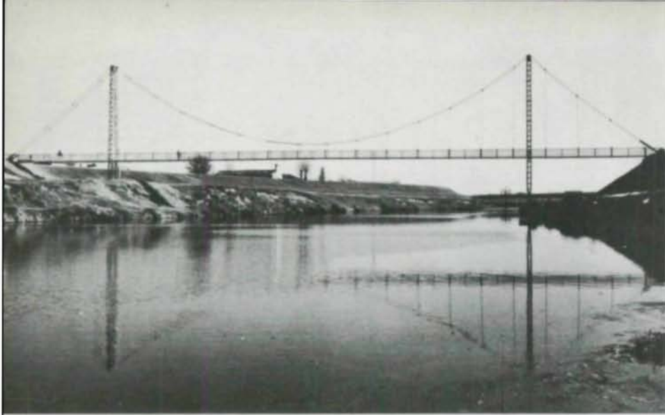
◀ Bridge Over the Brenta River, Padua, Italy For spans greater than 1200 ft, the steel suspension bridge may provide an economical as well as aesthetic pedestrian crossing.
