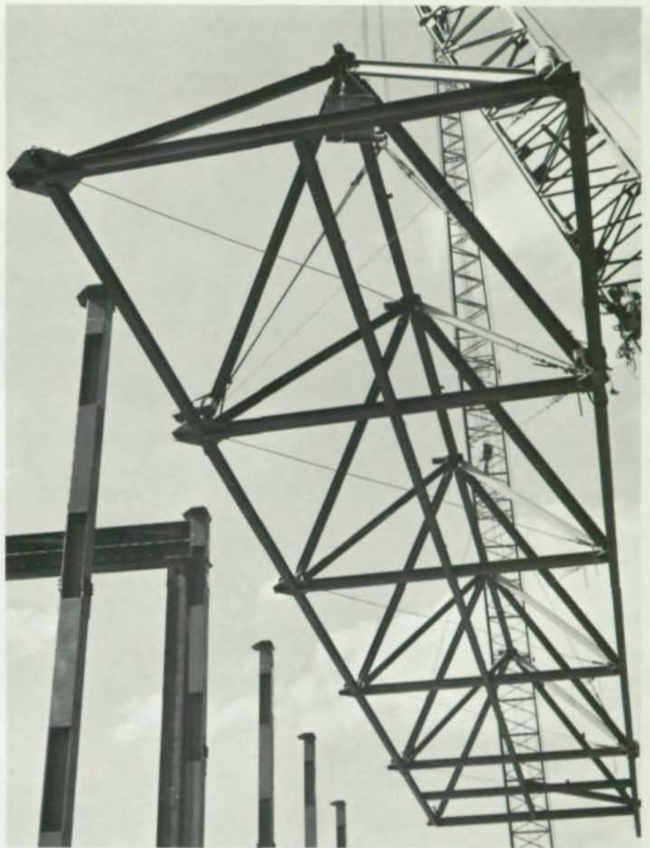
Subassemblies 150 ft long and weighing 40 tons were put together on the ground, then hoisted 80 ft above grade to be joined to supporting columns and to each other. Connections joined eight steel members, weighed ¾-ton each.
