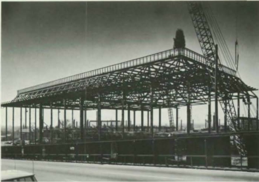
The huge roof is made up of 121 steel pyramids that act together as a single structural frame.
