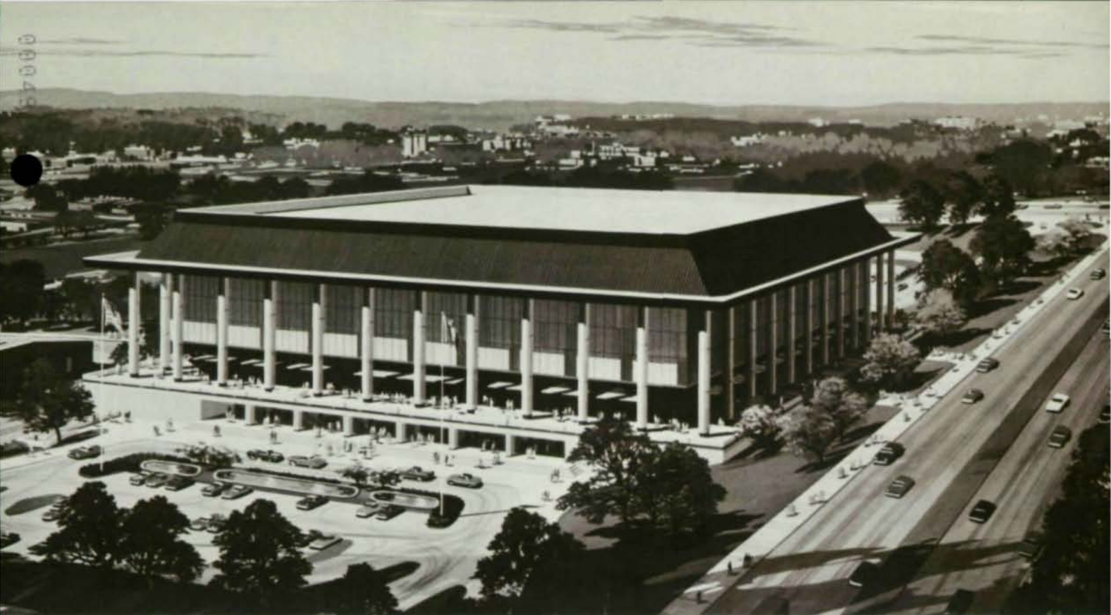
Largest academic-sports complex in the Southeast, the University of South Carolina Coliseum features a steel space frame roof spanning 322 ft x 322 ft between supports.
