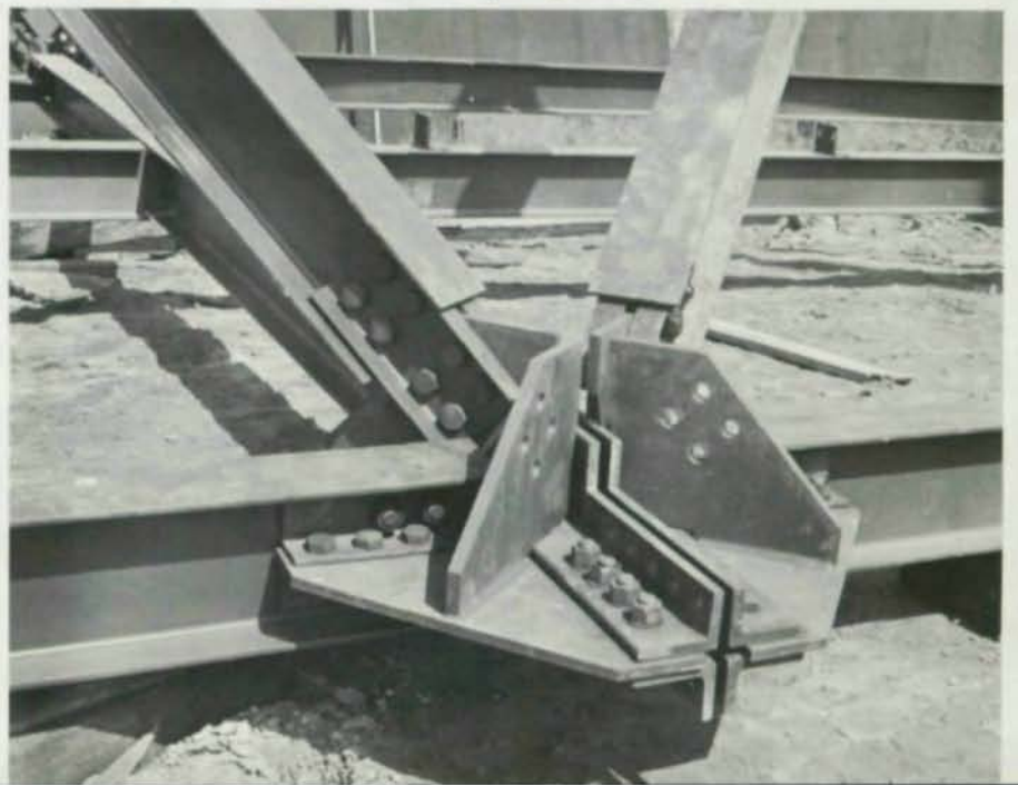
Subassemblies 150 ft long and weighing 40 tons were put together on the ground, then hoisted 80 ft above grade to be joined to supporting columns and to each other. Connections joined eight steel members, weighed ¾-ton each.
