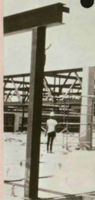
The two-way truss frame was assembled on the floor, then lifted into place as a single unit. Four cranes, one at each corner, easily handled the 34½-ton assembly. Bar joists between the trusses and outriggers to frame the roof overhang were installed later.
