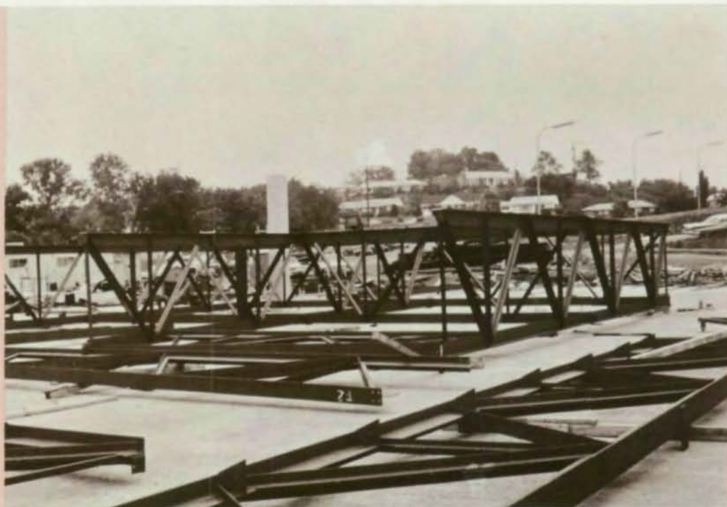
The two-way truss frame was assembled on the floor, then lifted into place as a single unit. Four cranes, one at each corner, easily handled the 34½-ton assembly. Bar joists between the trusses and outriggers to frame the roof overhang were installed later.
