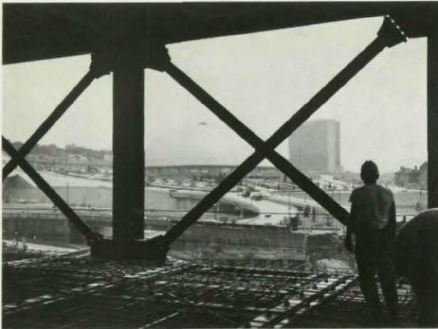
*Gap between column attachments and upper ends of X-brace members helps prevent "deformation" of members in the event framework is subjected to unusually severe horizontal loads.*
