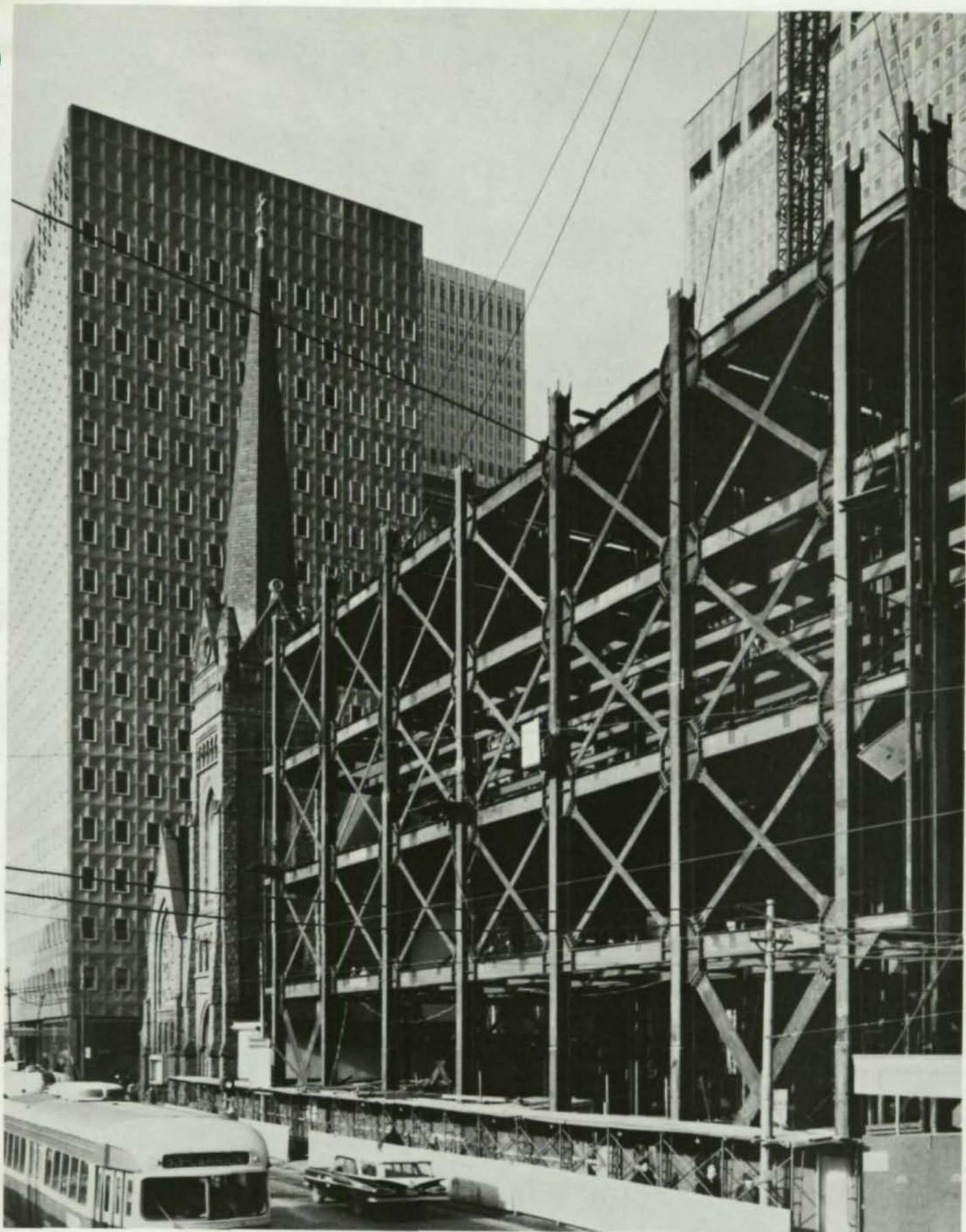
*Use of X-bracing members (ASTM A514 — 100,000 psi yield strength) reduced drift to a minimum.*
