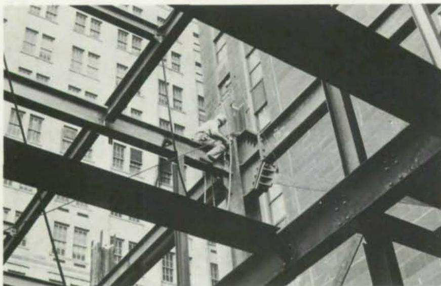
Ironworker arc welds high-strength steel "jumbo" column (730 lbs per sq ft).
