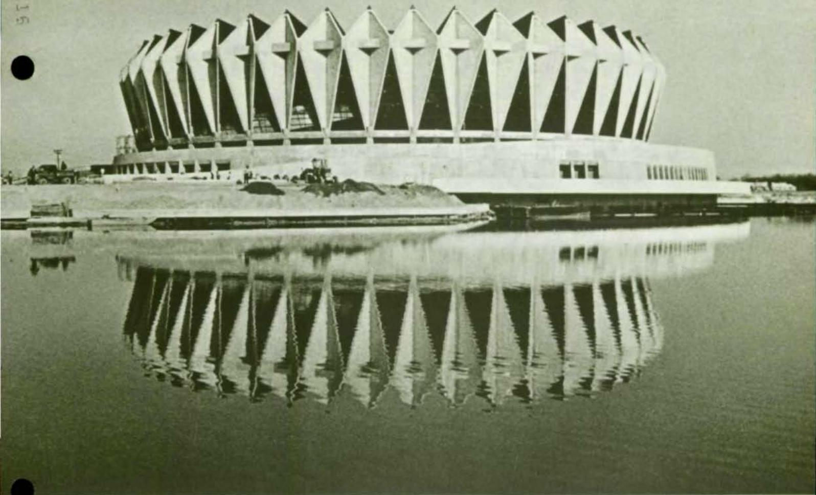
The design of the recently dedicated \$6.8-million Hampton Roads Coliseum, in Hampton, Va., was inspired by the symbol of the Tidewater area — white sails. Exterior sail-shaped wall panels support a 400-ft dia. cable-suspended clear span roof.
