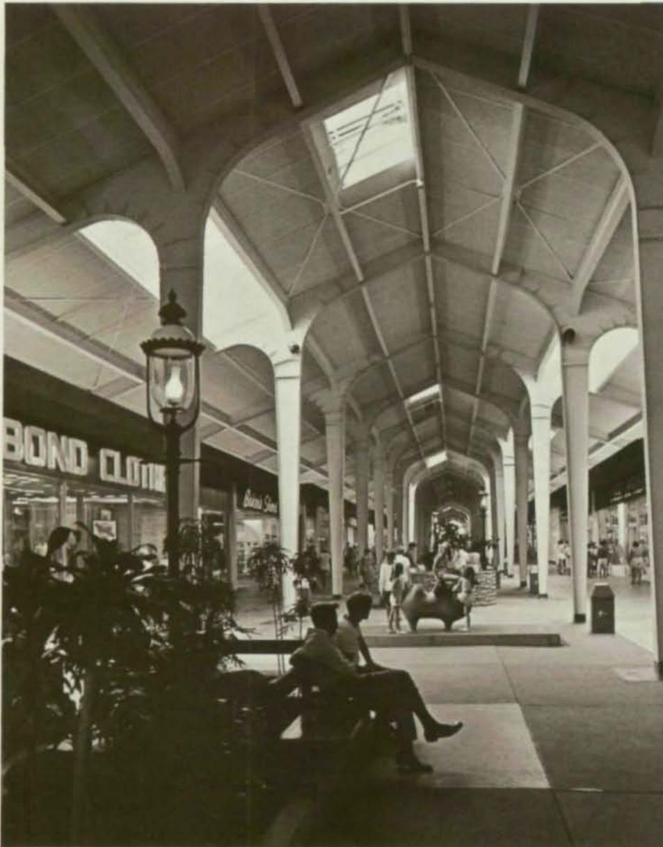
The design of the bents achieves a high spacious volume through the center of the mall and creates more intimate walkways of comfortable scale along the storefront shopping areas. Skylights are used intermittently to form pools of daylight and various light intensities for interest and accents.
