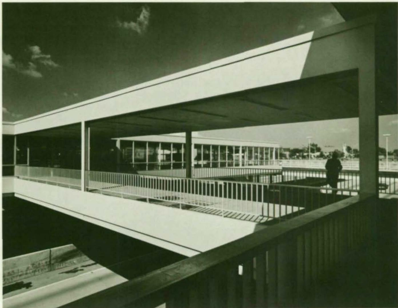
posed by structures of these types. Welded steel connections were used to give a finished appearance, and to obtain smooth surfaces. Finally, the architects were able to make the steel construction the basis of the architectural expression of the stations, since the building code permitted non-fireproofed steel in most cases.
