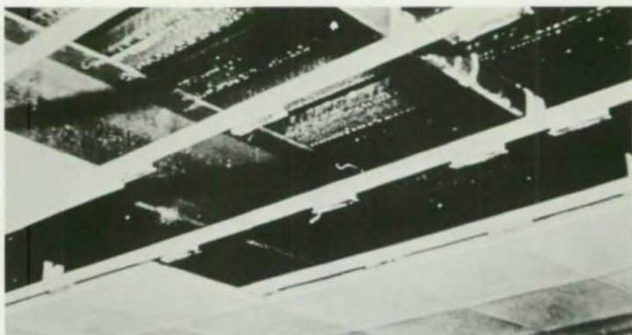
*Fire-rated acoustic tile ceiling showing exposed steel decking and beam*
