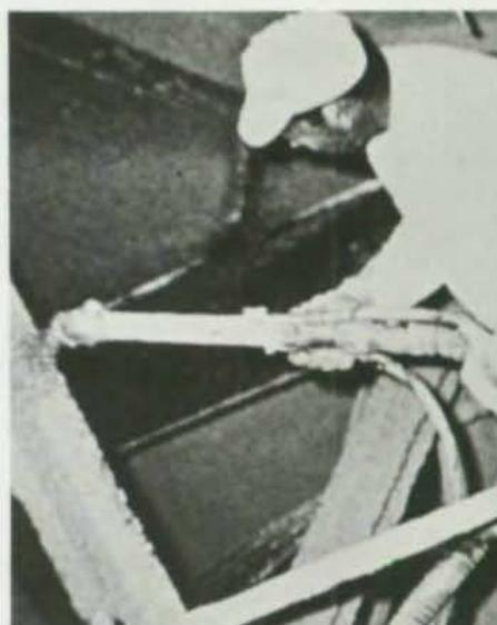
*Application of sprayed protection*
