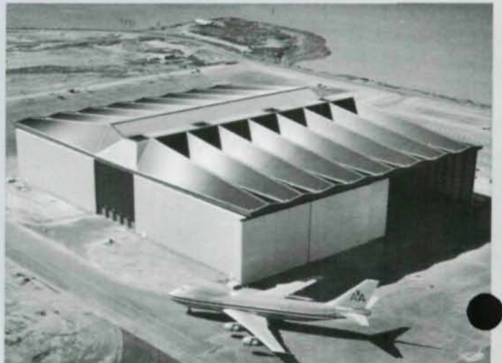
▼ SUPERBAY MAINTENANCE FACILITIES San Francisco International Airport, San Francisco, Calif. Los Angeles International Airport, Los Angeles, Calif. Architect: Conklin & Rossant, Architects
