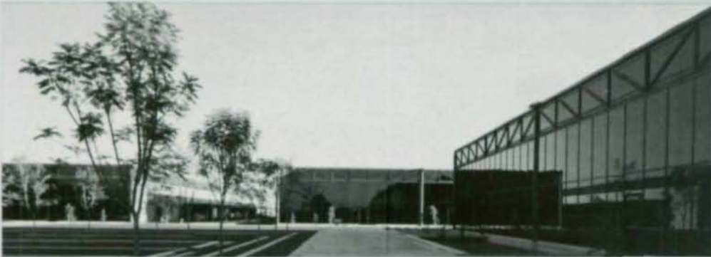
▲ PARKER HANNIFIN CORPORATION IRVINE FACILITY Irvine, California Architect: Albert C. Martin and Associates
