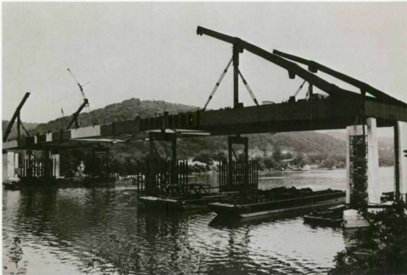
Fig. 9.—Glenfield Bridge, rib erection
