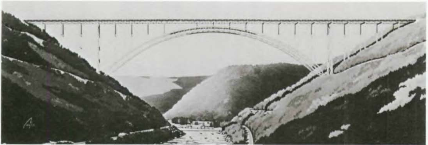
Fig. 10.—New River Gorge Bridge
