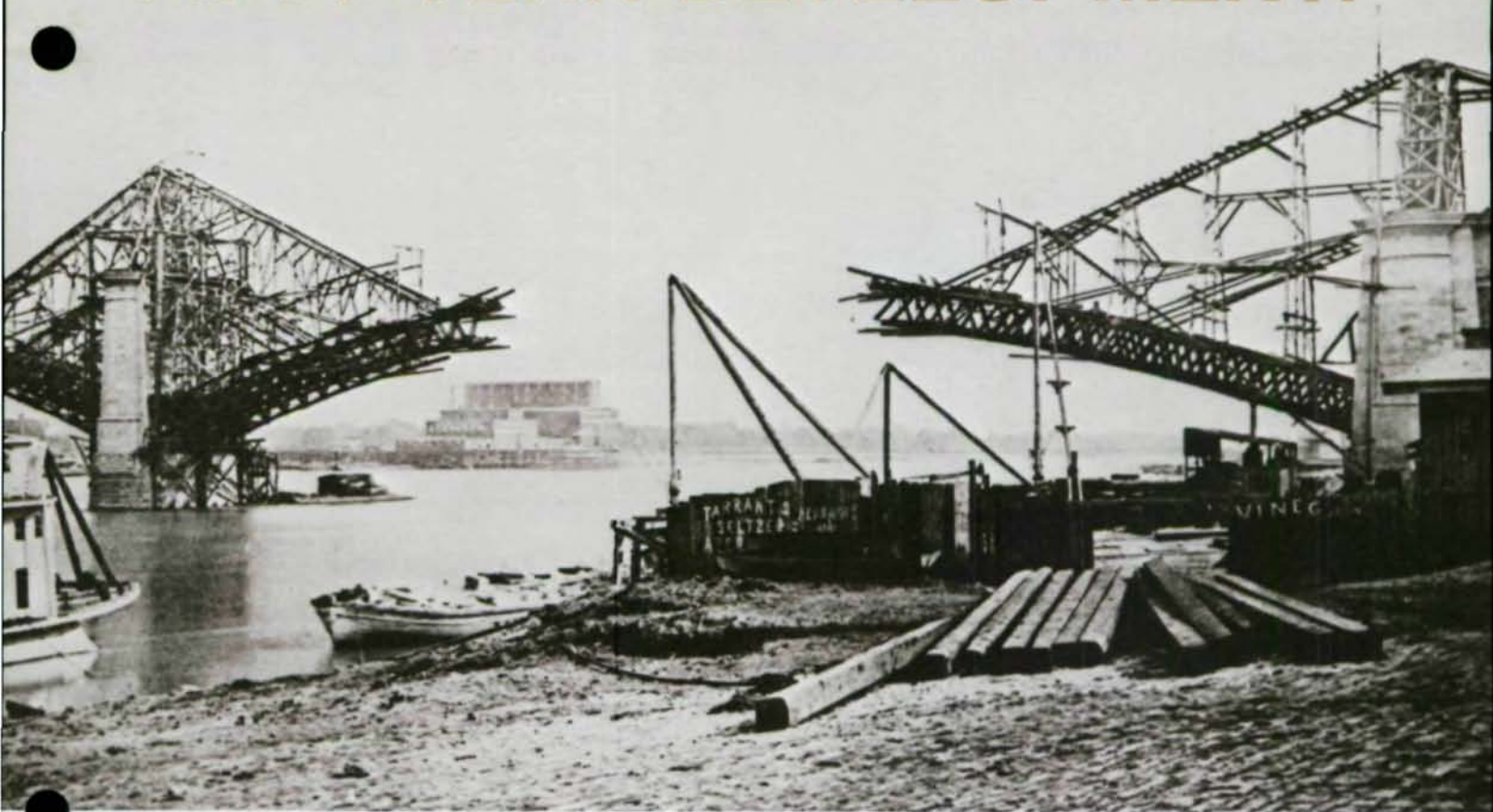
Fig. 1.—Eads Bridge, erection with tieback cables (Courtesy of Joseph E. Vollmar, Jr.)
