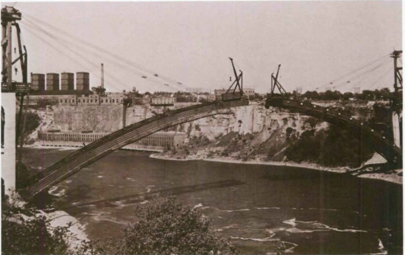
Fig. 5.—Rainbow Bridge, erection by traveler (Courtesy of Bethlehem Steel Corporation)
