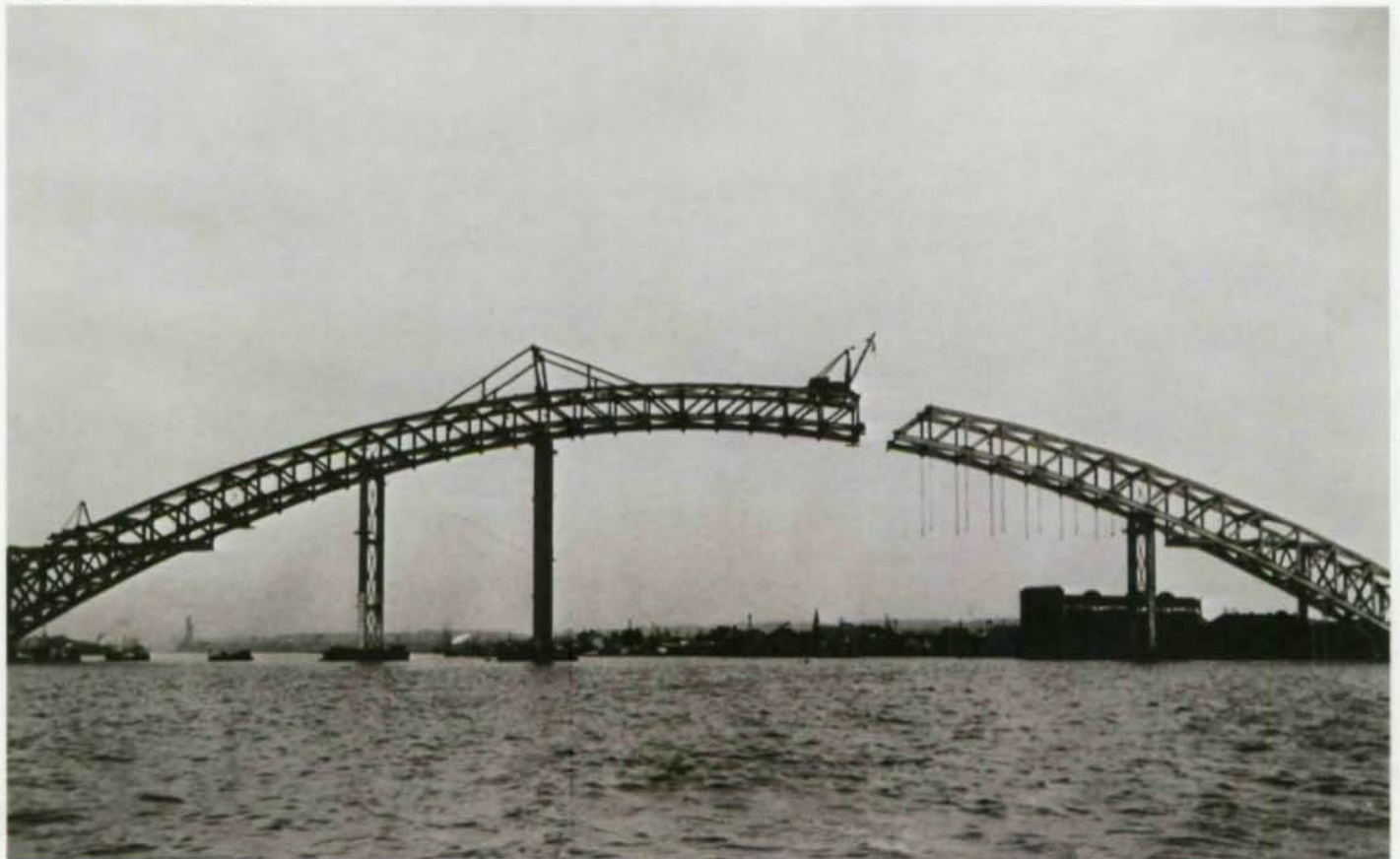
Fig. 3.—Bayonne Bridge, arch nearing closure
