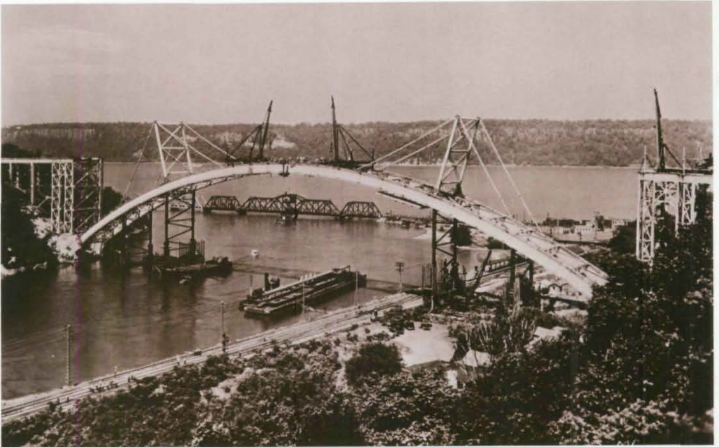
Fig. 4.—Henry Hudson Bridge, arch after closure
