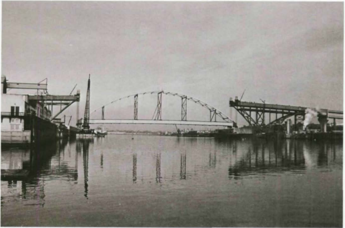
Fig. 8.—Fremont Bridge, lifting of arch span
