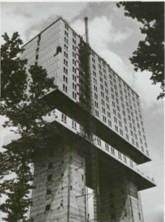
Sixteen synchronized hydraulic jacks (tied into a central console) lifted each floor at the rate of 15 ft per hour.
