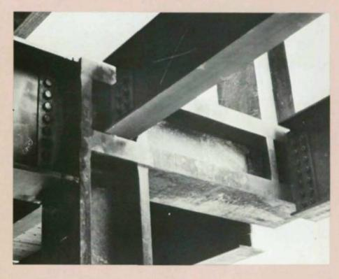
Mechanicals for the many energysavings systems to be tried in the building can be accommodated more easily by the steel framing system since framing members are reduced in thickness as compared to a possible concrete design.
