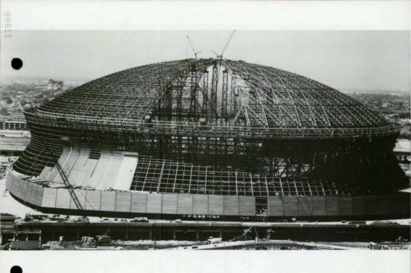
ing each radial bent as a braced, rigid frame. The New Orleans Building Code specifies 60 psf above 100 ft which is comparable to a 153 mph wind. Wind analysis was based on a wind study using a scale model (1 in.: 24 ft). The shape of the Superdome resulted in nearly all roof and wall pressures being negative or uplift. The ICES STRUDL computer system was employed for the structural analysis. The final roof system required 26 psf of structural steel.
