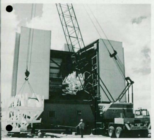
Subassemblies of the Optical Support Structure (OSS).
