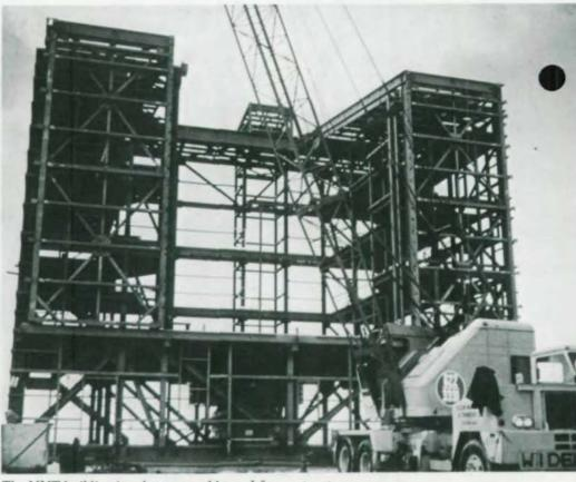
The MMT building is a 4-story steel braced frame structure.
