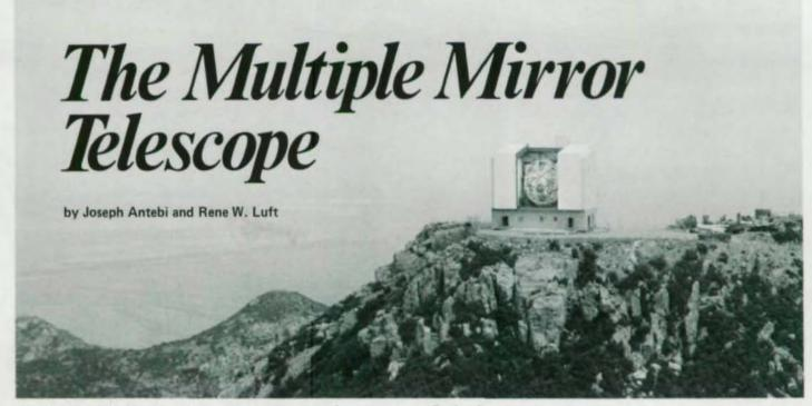
Perched atop Mt. Hopkins, the entire telescope complex rotates on a flat hardened-steel track.
