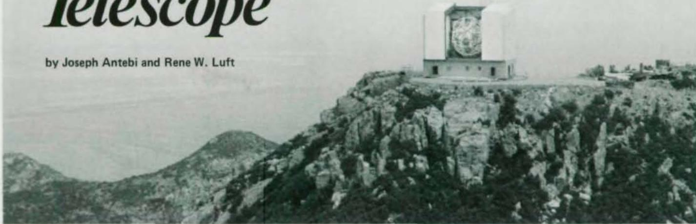
*Perched atop Mt. Hopkins, the entire telescope complex rotates on a flat hardened-steel track.*
