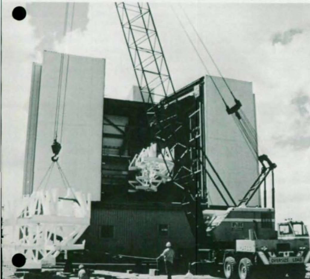
Subassemblies of the Optical Support Structure (OSS).
