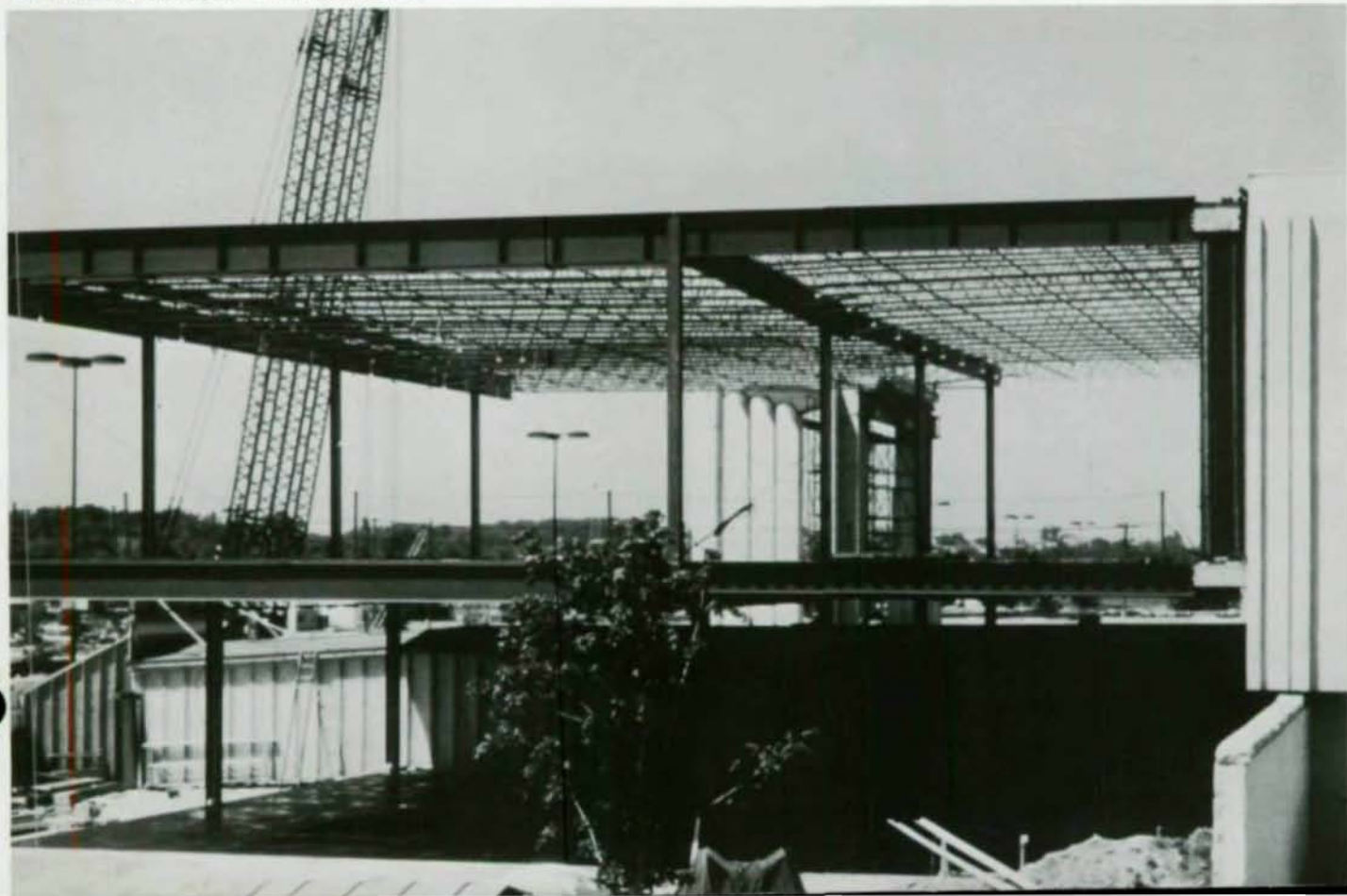
Original Boston Store's concrete-framed building was enlarged with steel-framed addition at considerable savings in both cost and time.
