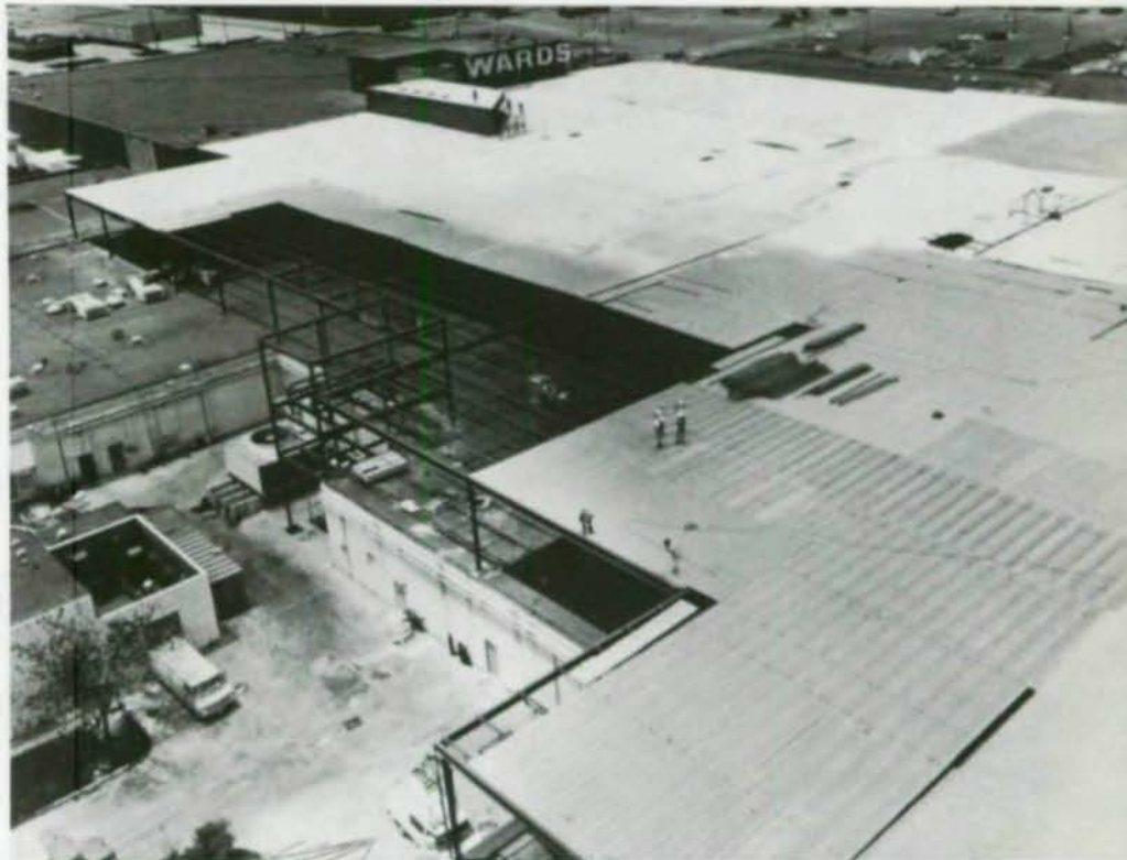
Roof goes on over new addition before old one was removed. Airconditioning and skylight units also remained in place until building was enclosed.
