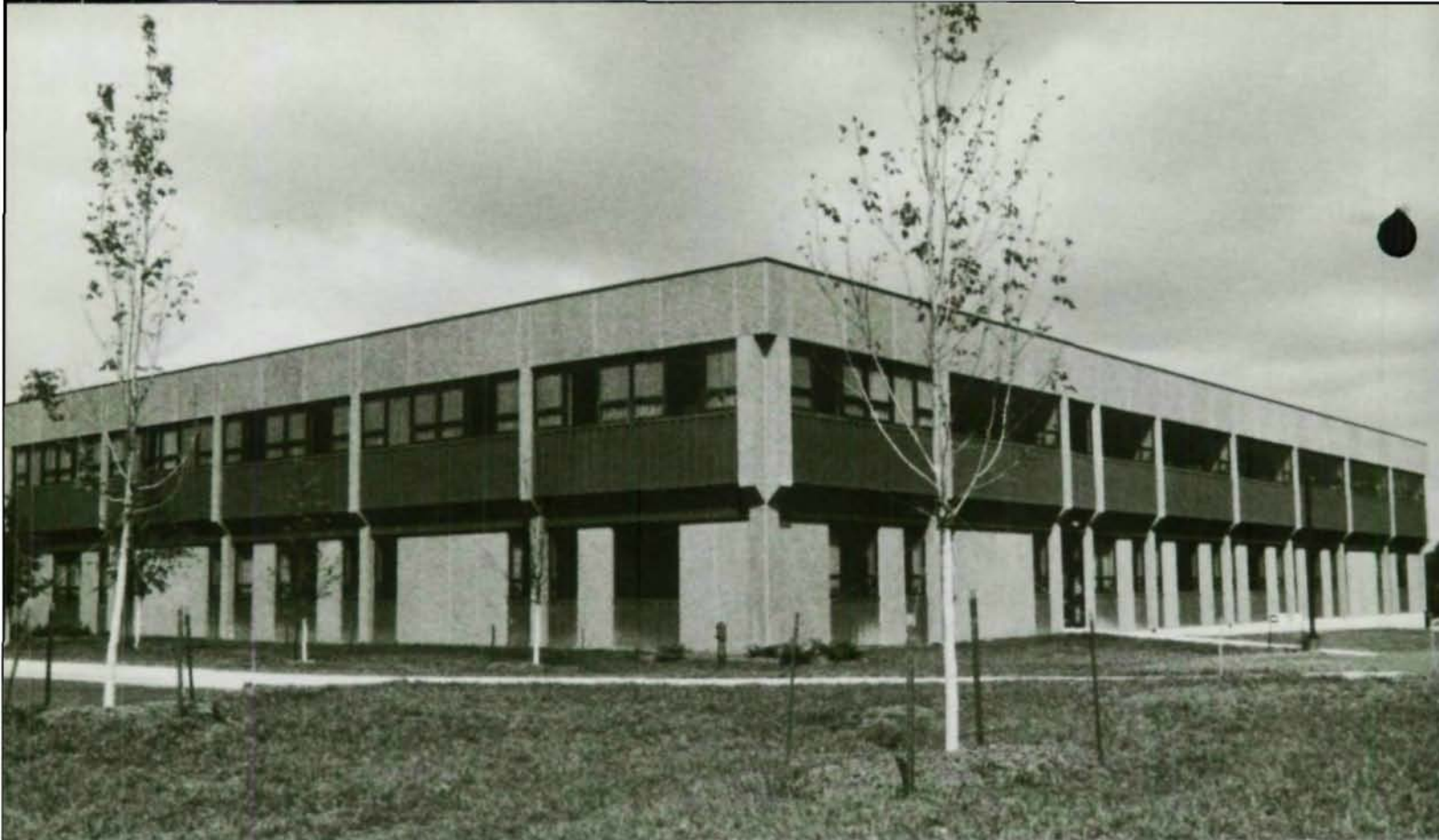
Simmonds Precision Products' new headquarters in Vergennes, VT. Million-dollar change order added second story to building already under construction. Drawing (next pg.) details steel construction that speeded progress.
