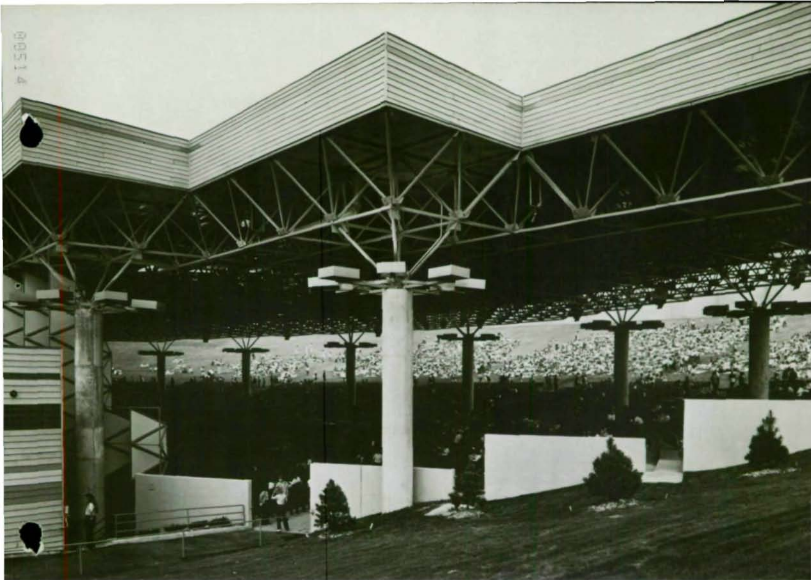
Poplar Creek Music Theatre, Hoffman Estates, IL is largest of its kind. Steel-tube space frame bears on 42-in. concrete columns. Its 60,000 sq ft (below) shelters 7,000 people indoors. View towards lawn seating area.
