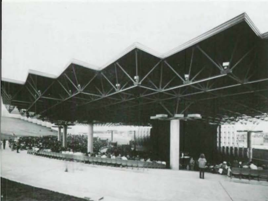
Looking toward stage and lawn seating area (bottom). Radiating uplifts on columns hold house lights. Space frame and roof deck underside are painted bright red, add festive air by reflecting floodlights. Note sound barrier walls in background.
